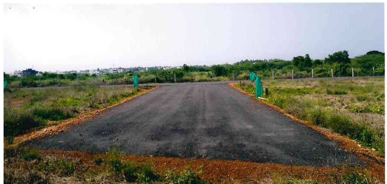
E Boundary - W Facing Road 2-2
