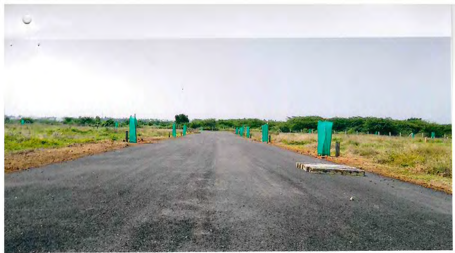
E Boundary - W Facing Road 3-3
