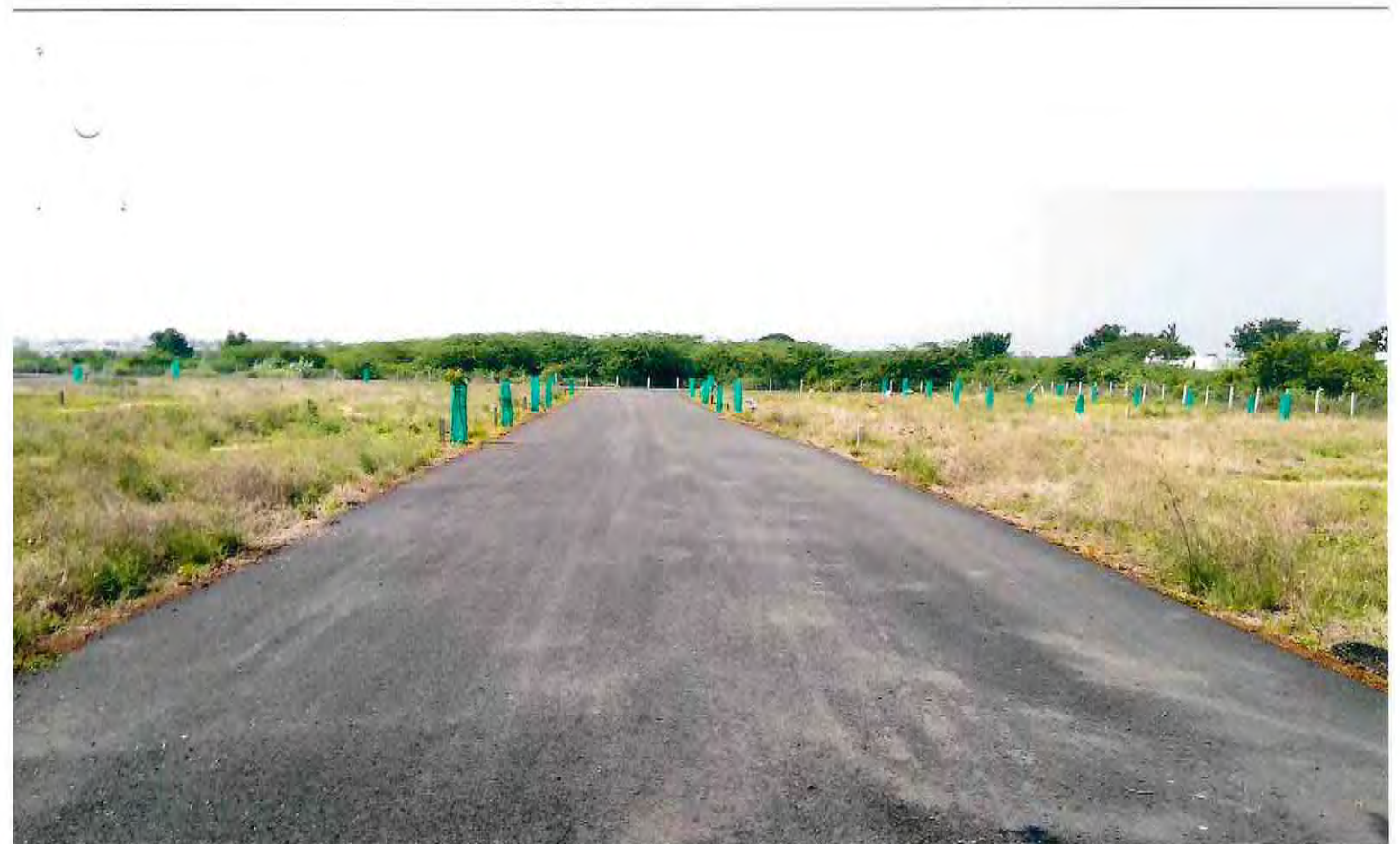
E Boundary - W Facing Road 4-4
