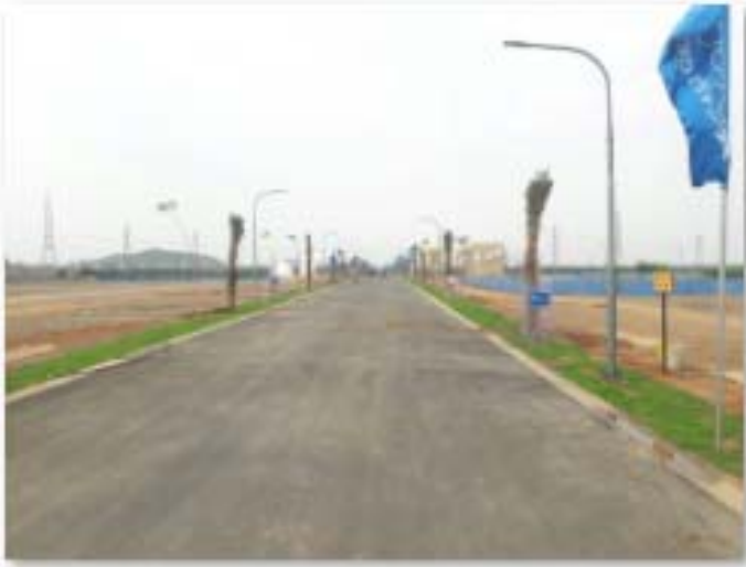
Road work completed
