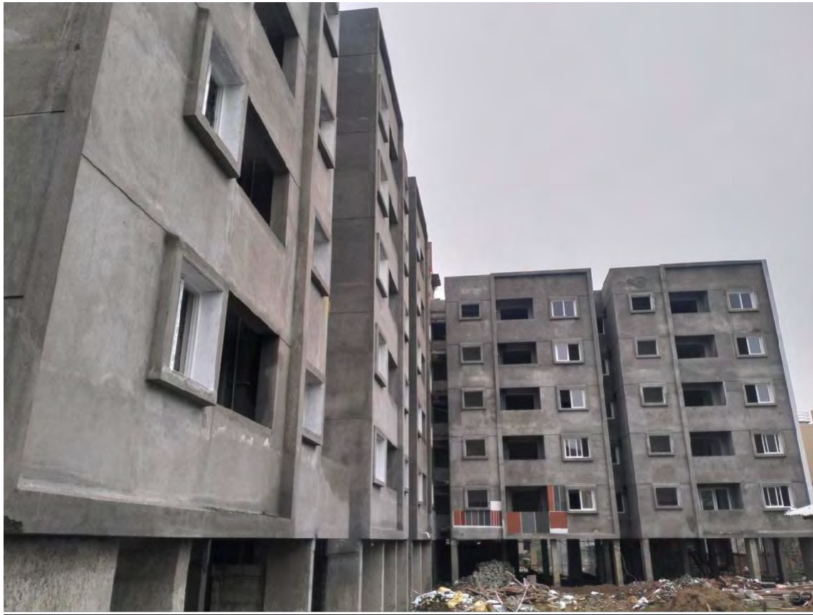
Block – B: Internal, External Plastering and Flooring work in progress
