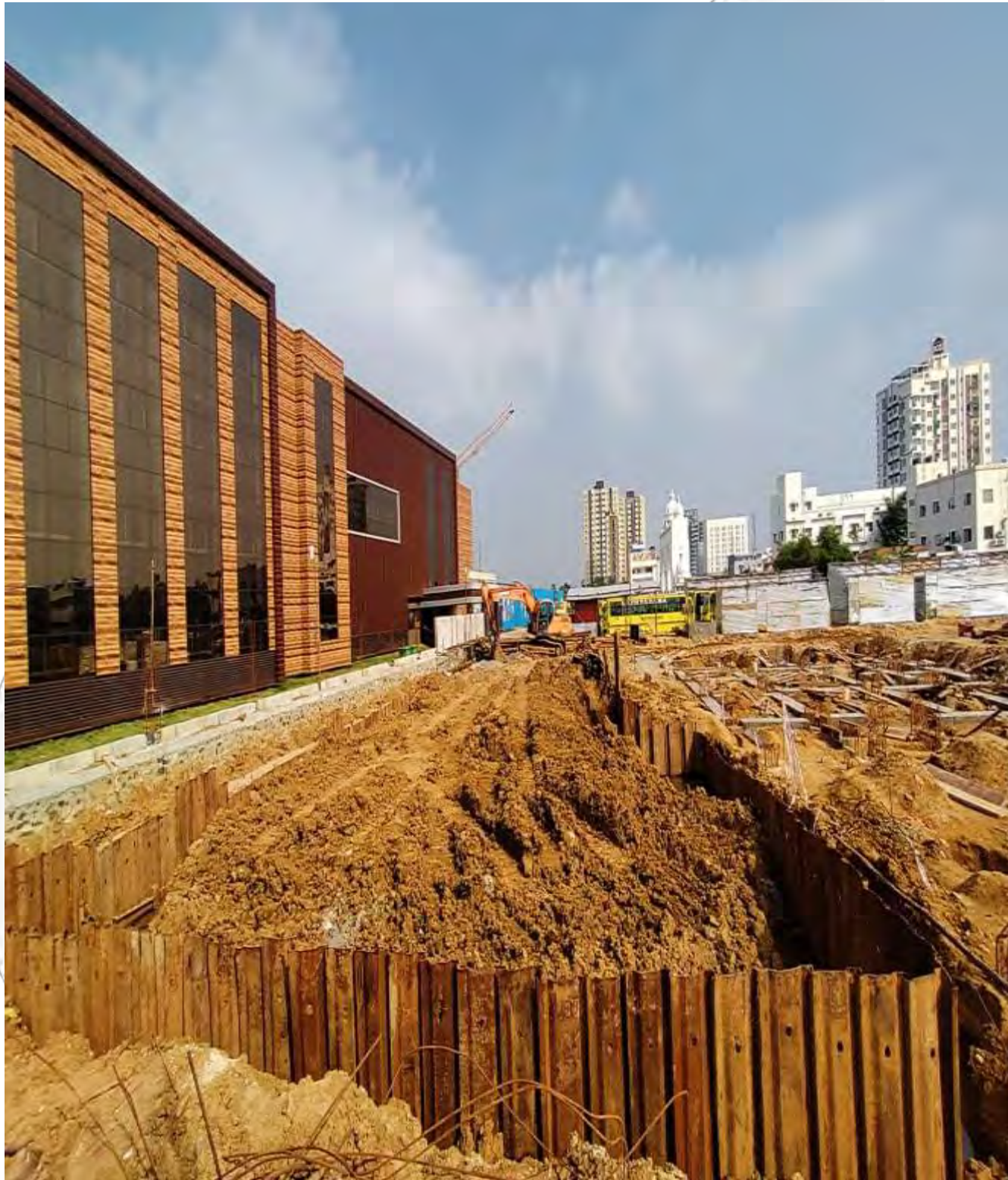
Block 1 - STP Shoring Works In Progress
