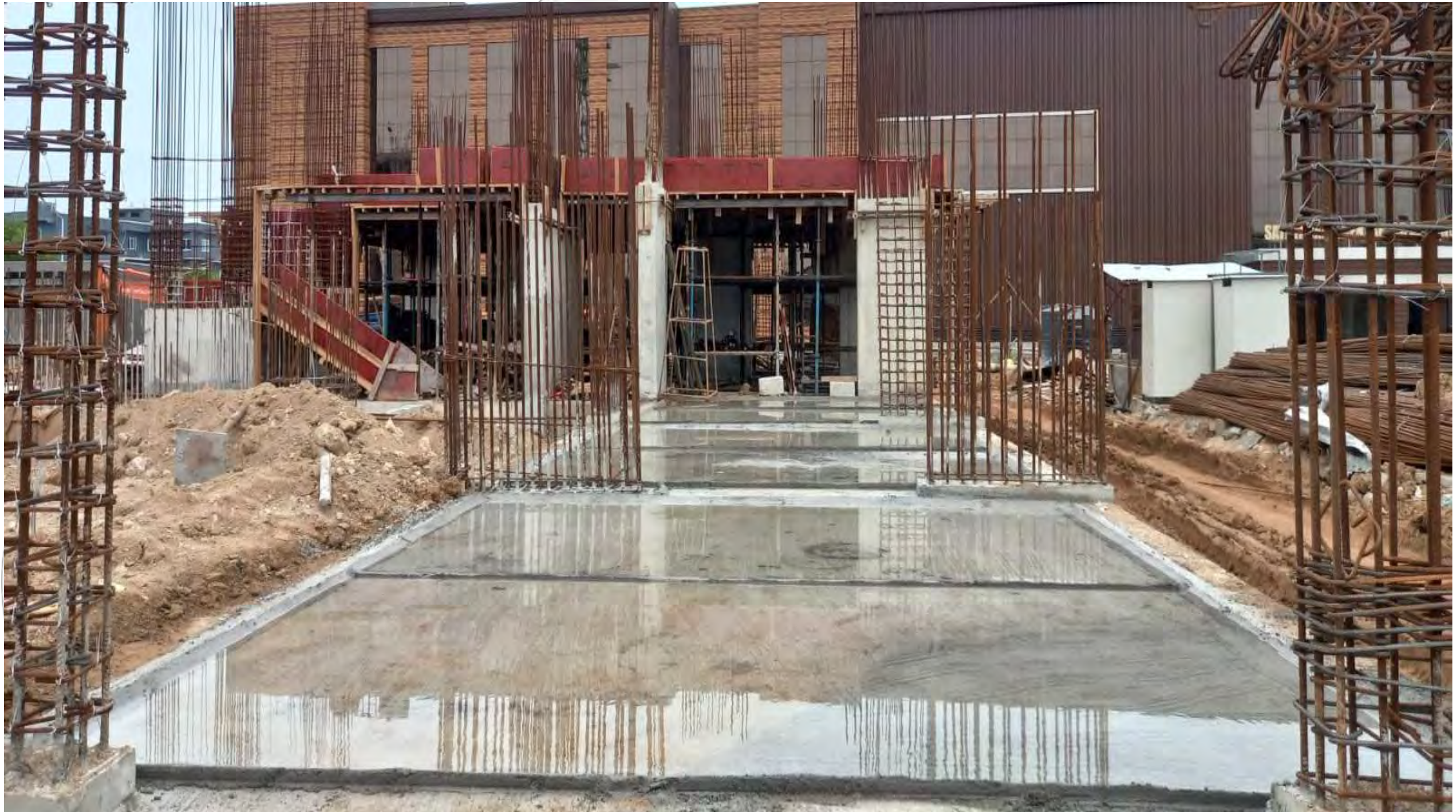
BLOCK 2 – STILT FLOOR PCC (POUR 1) IN PROGRESS.
