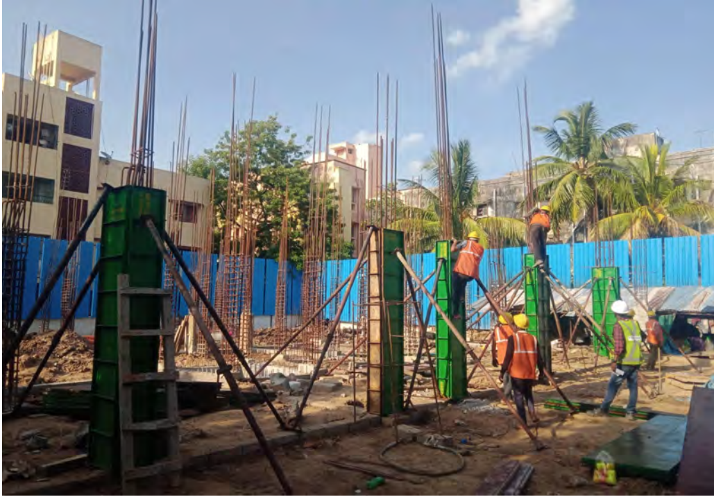
Column 2nd Lift Shuttering works
