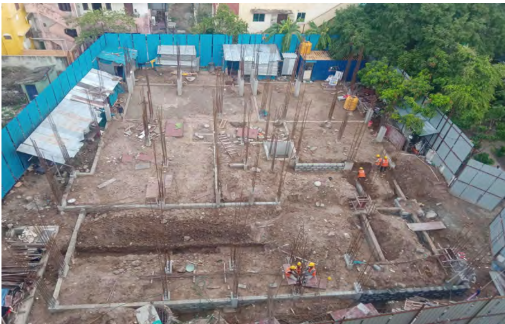
Pile Cap & Plinth beam 100% casting Completed.
