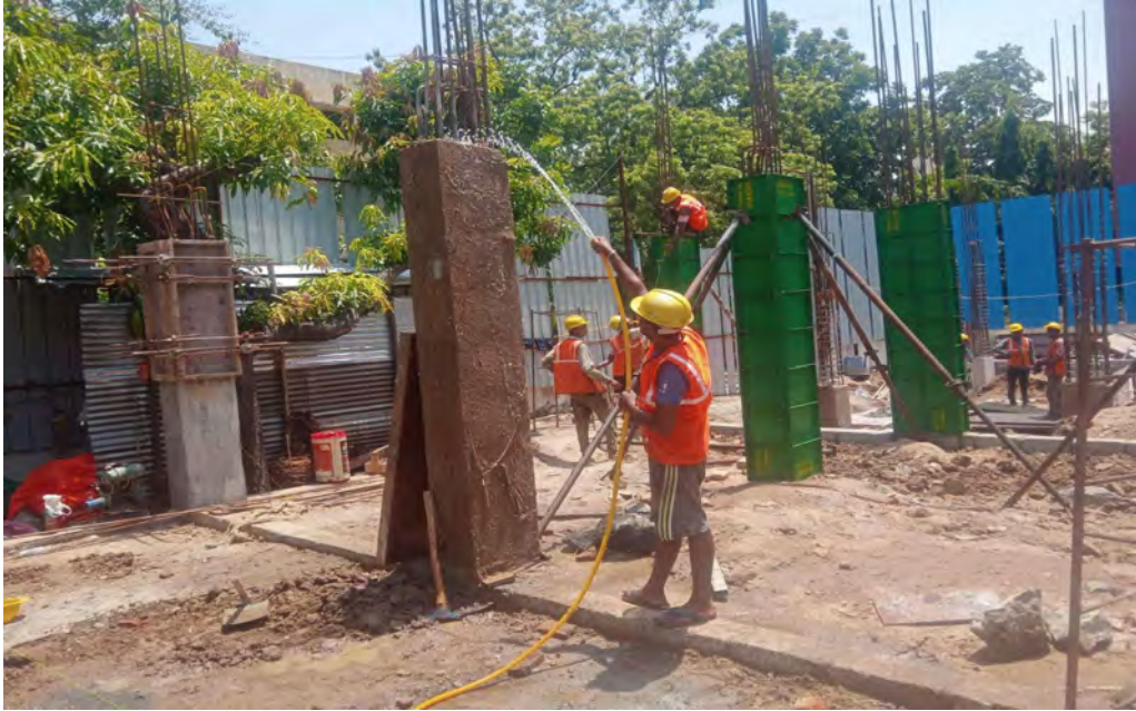
Column Curing Works
