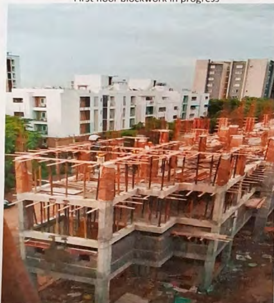
Third Floor Roof Beam shuttering in progress
