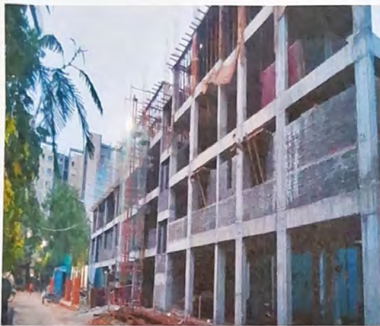
First floor blockwork in progress
