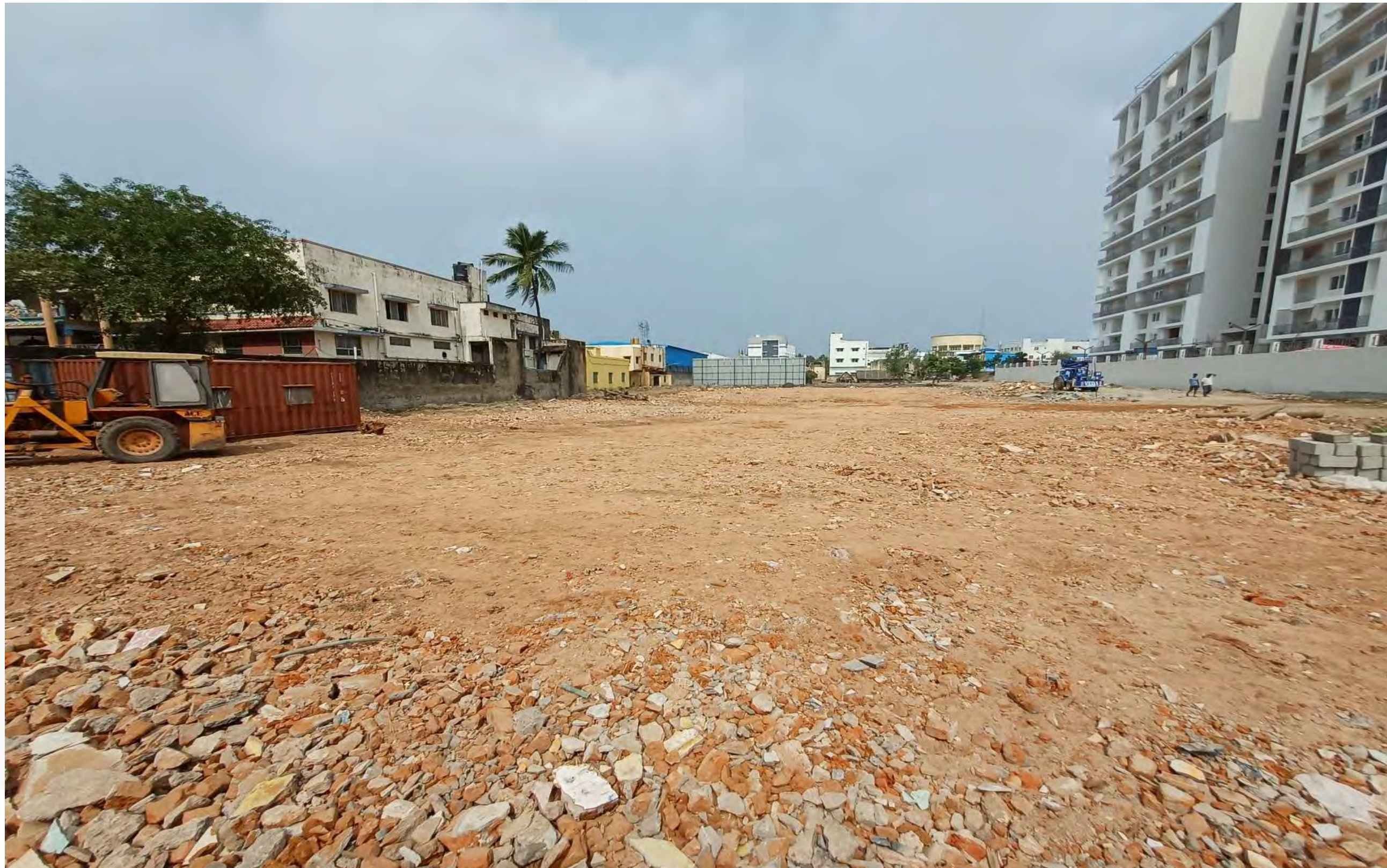
Base Preparation Works In Progress
