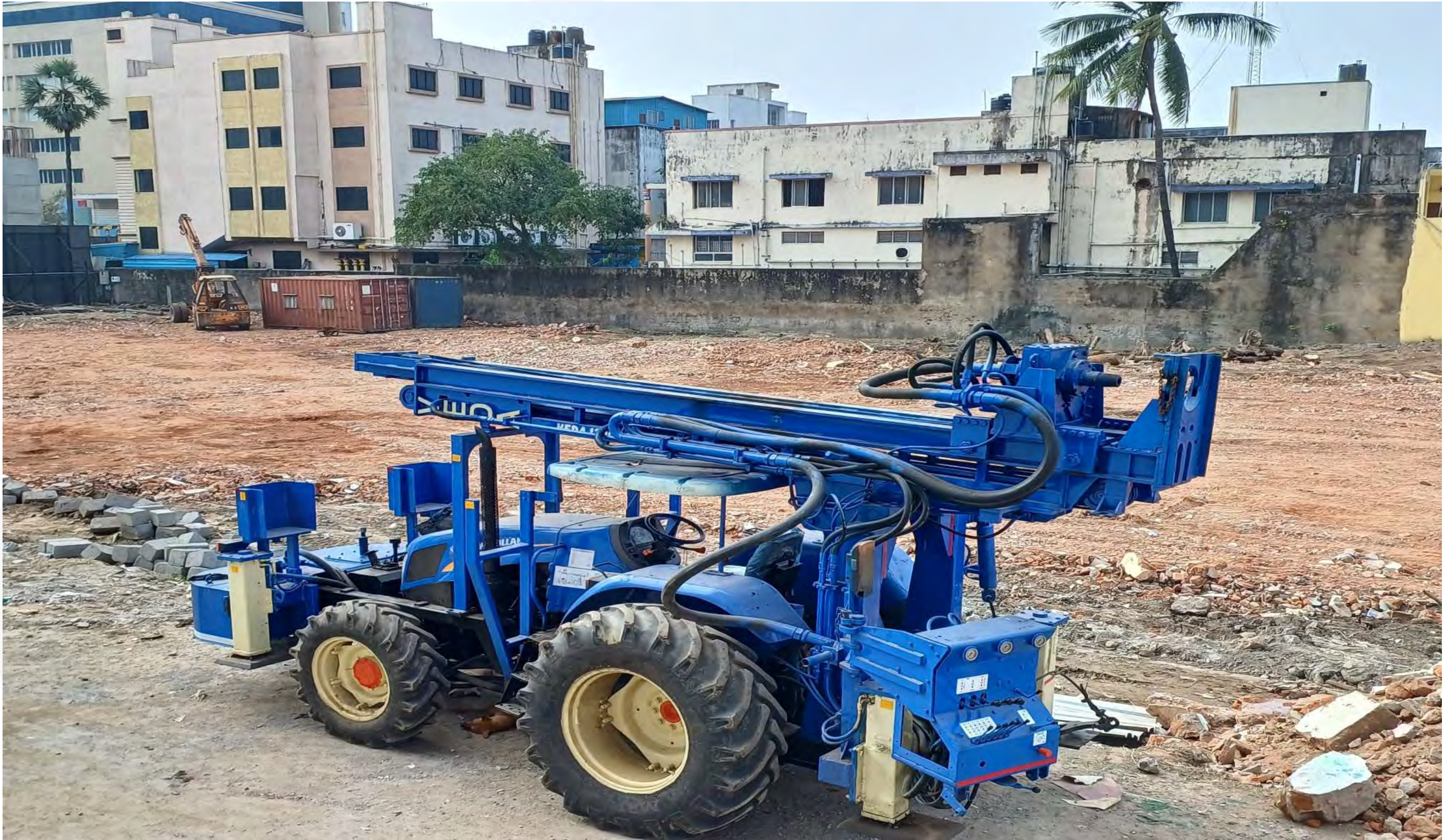
Pile Mobilization Work In Progress
