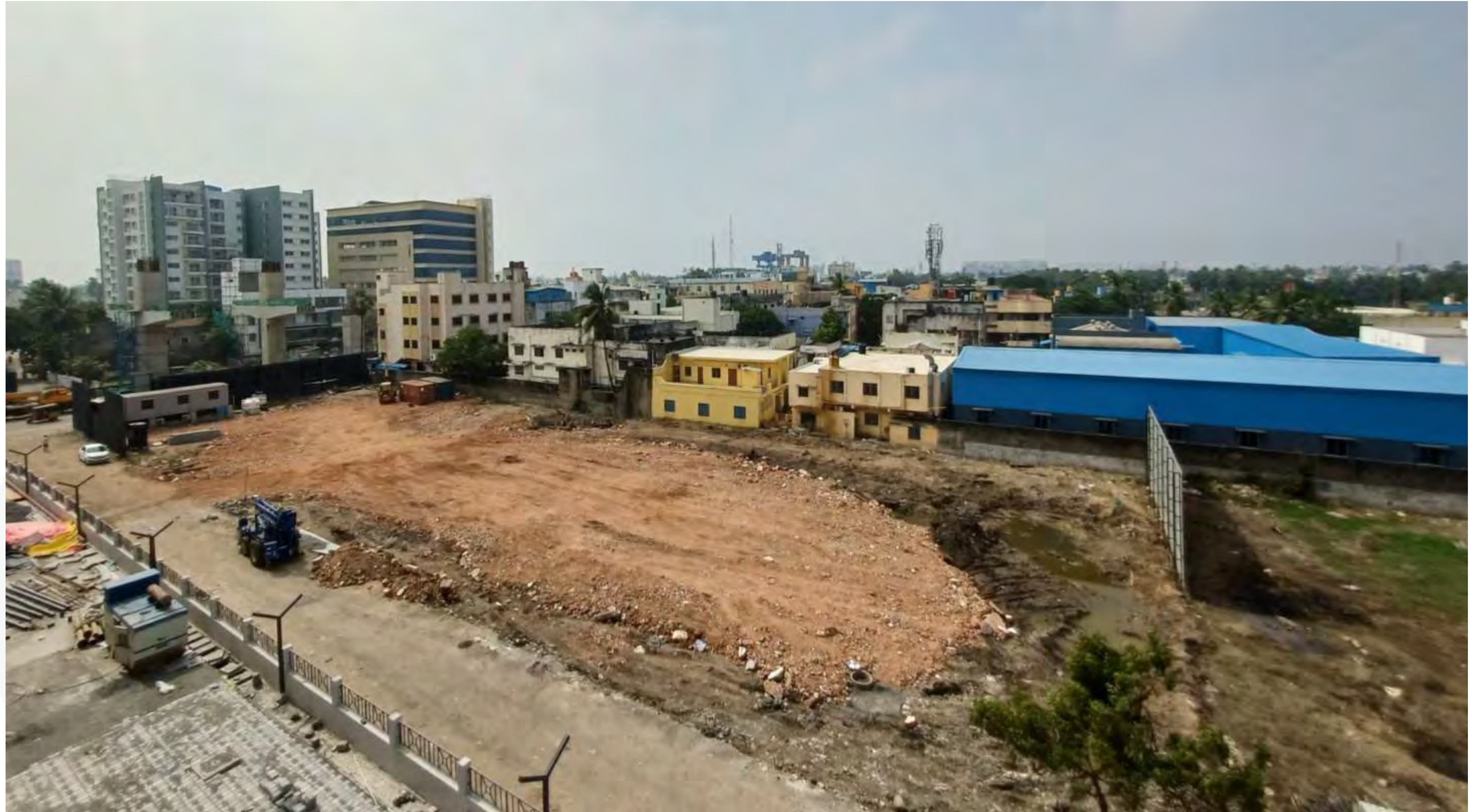
Base Preparation Works In Progress
