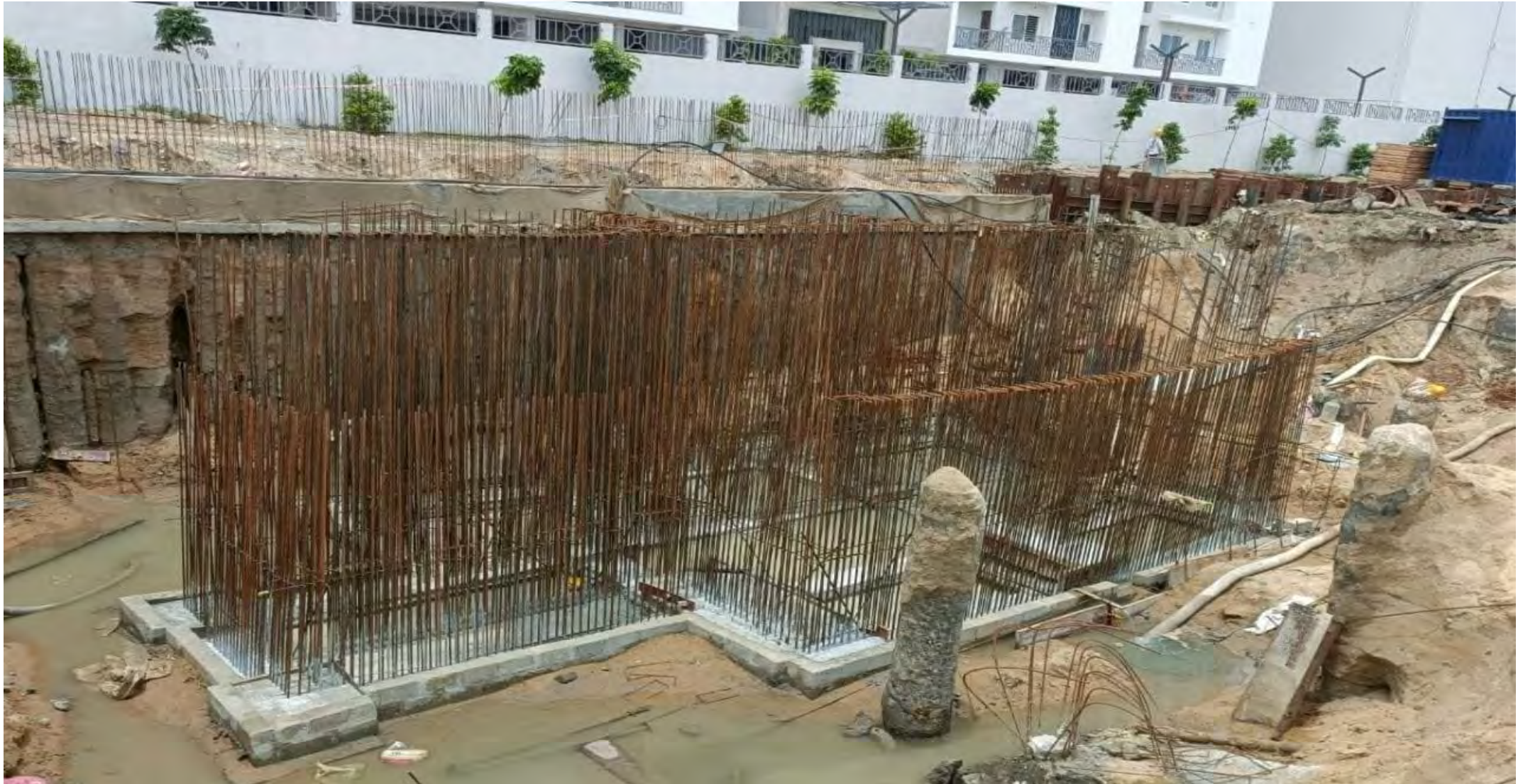
STP Raft Concrete Pouring Work Completed.
