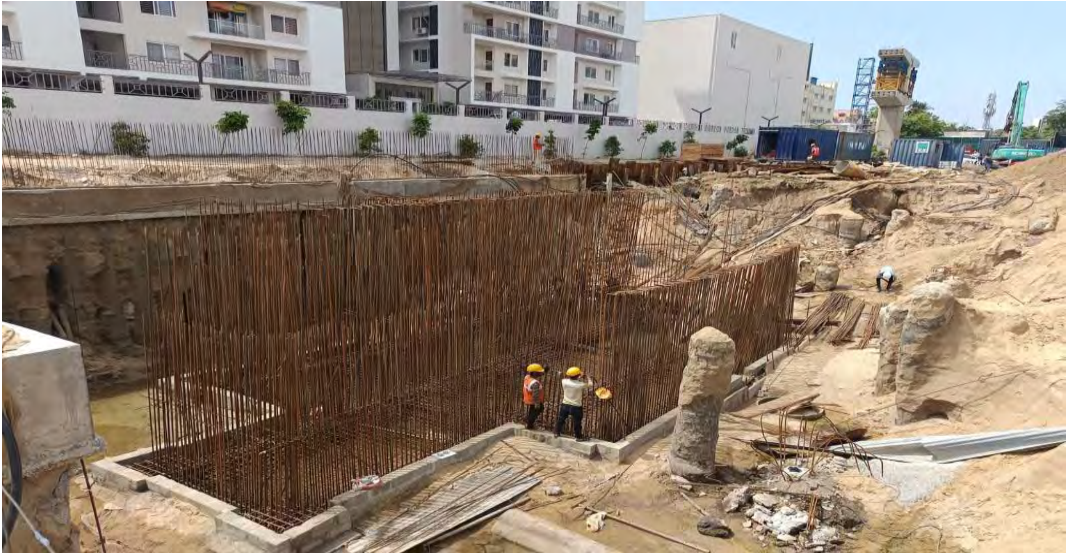
STP Raft & Wall Reinforcement Work Completed.
