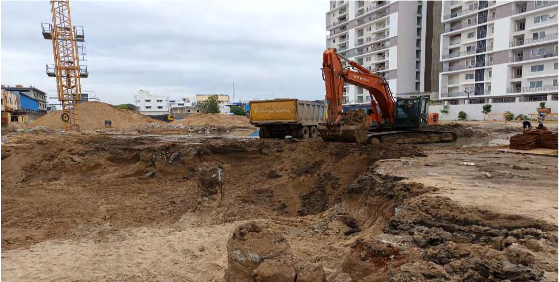
Excavation Work in Progress.
