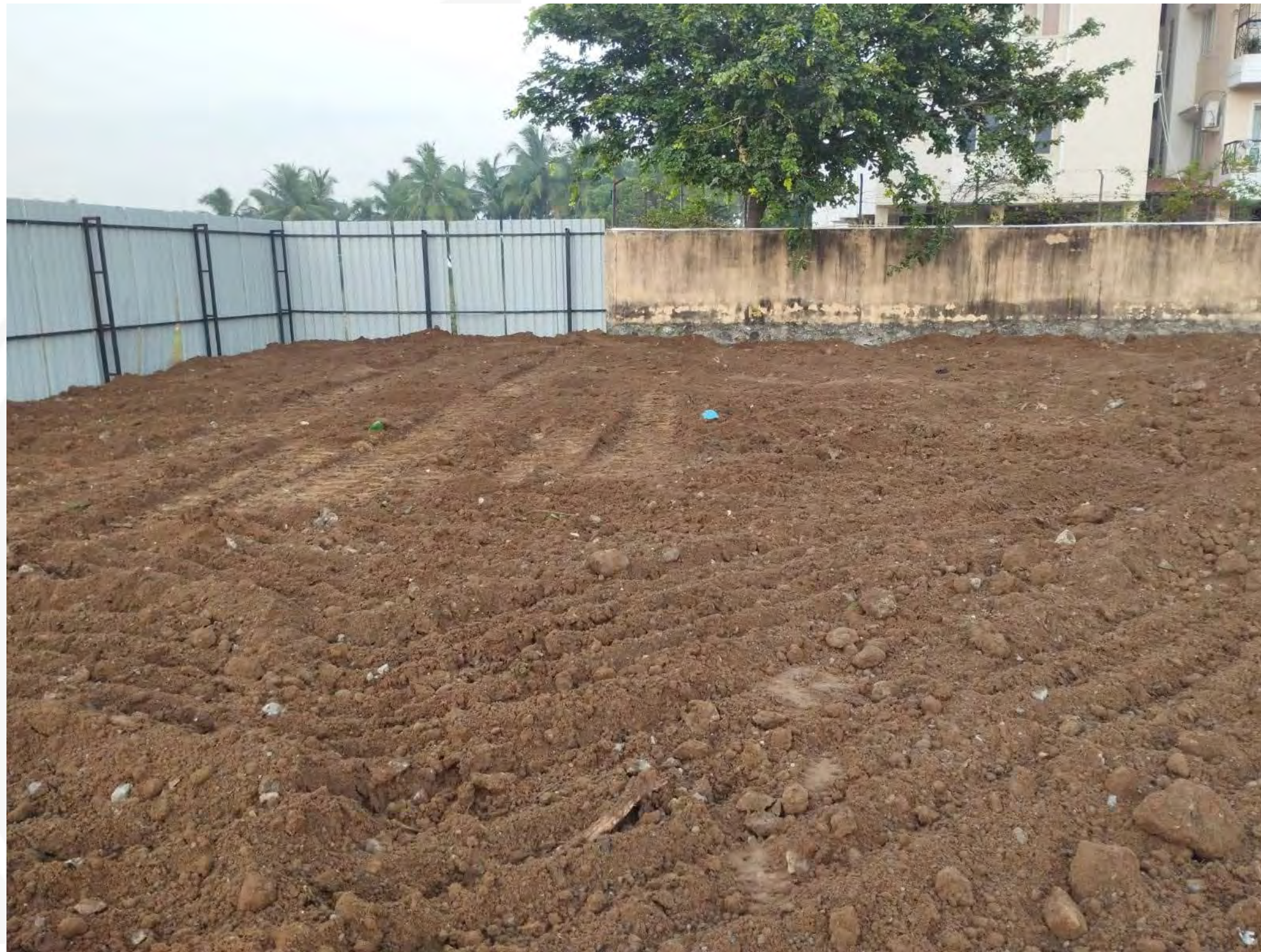
Earth Filling Work In Progress
