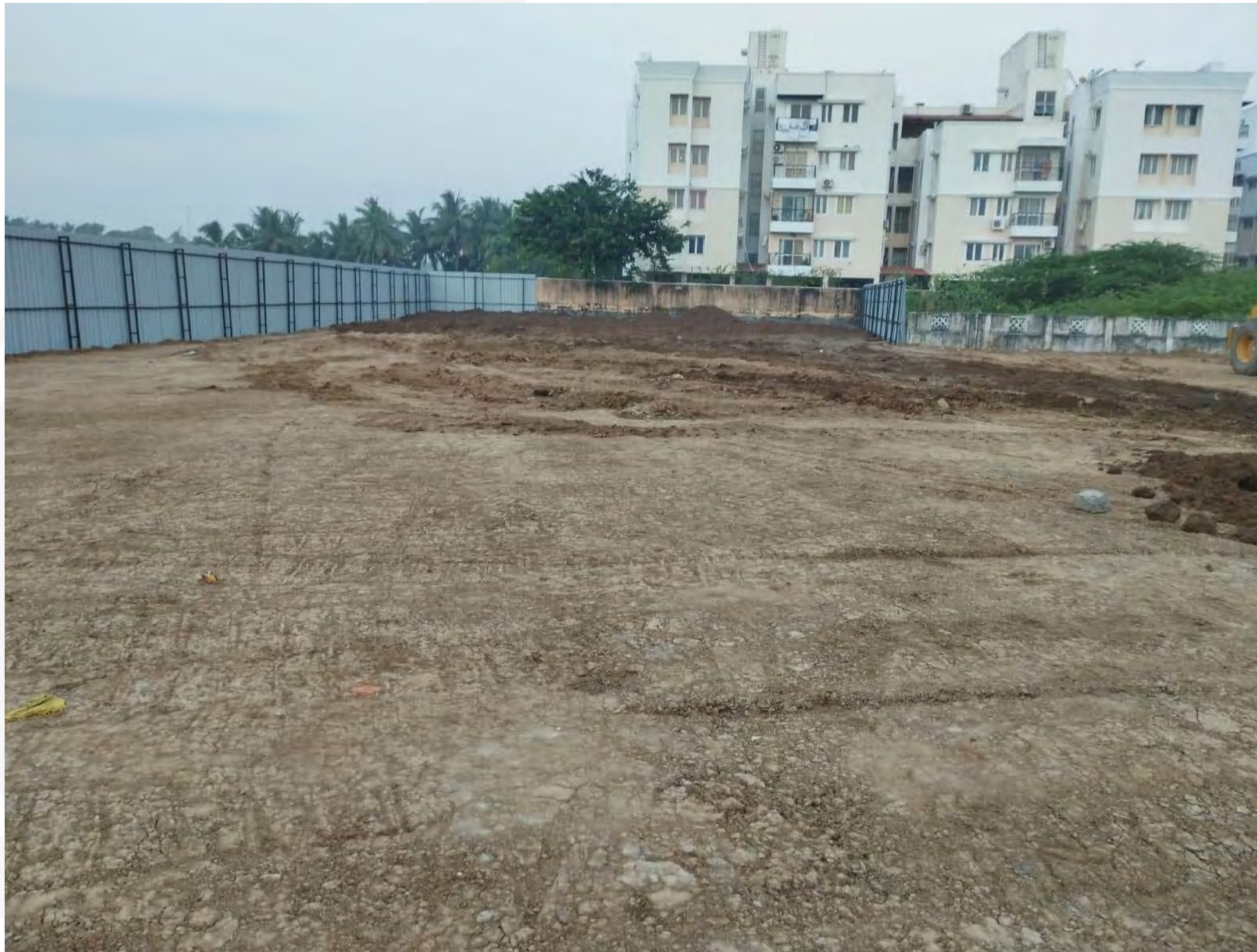
Earth Filling Work In Progress
