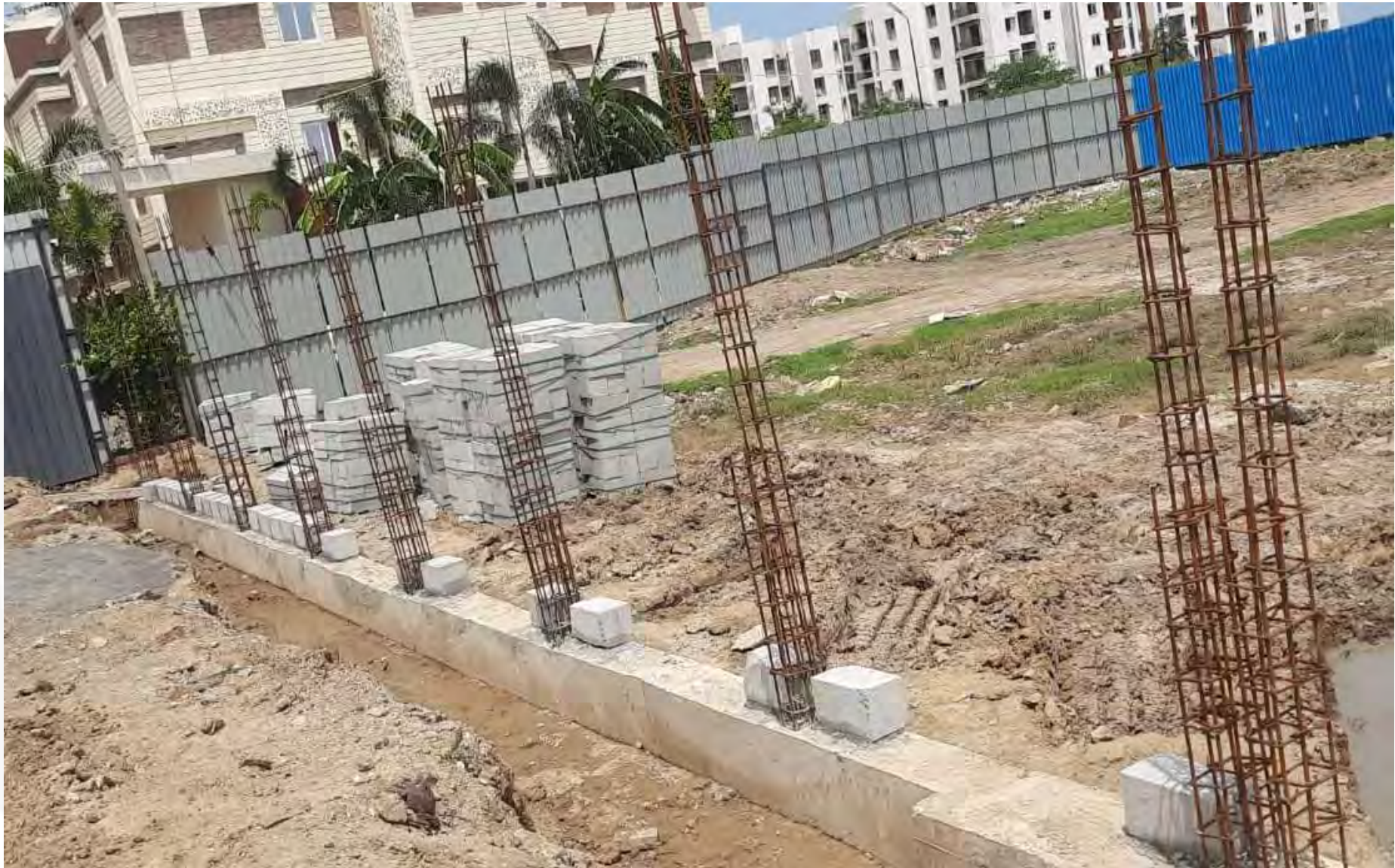
Compound Wall Blockwork Work in Progress.
