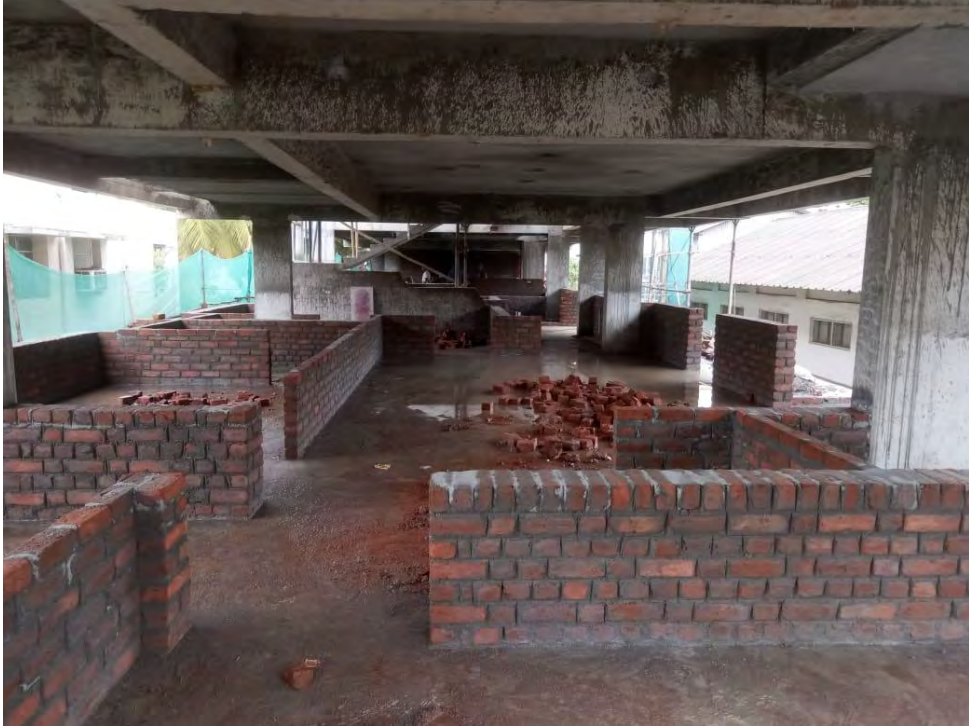
BRICKWORK
