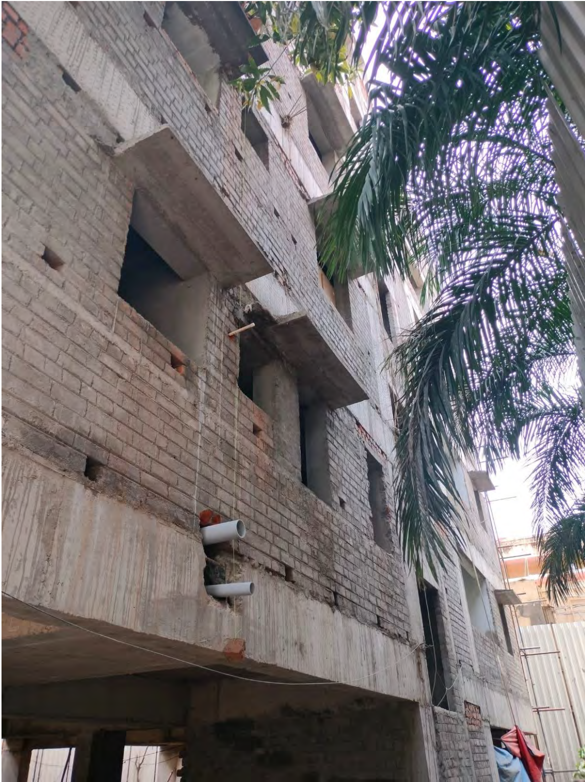
Site Conditions Photos : ( East side View )
