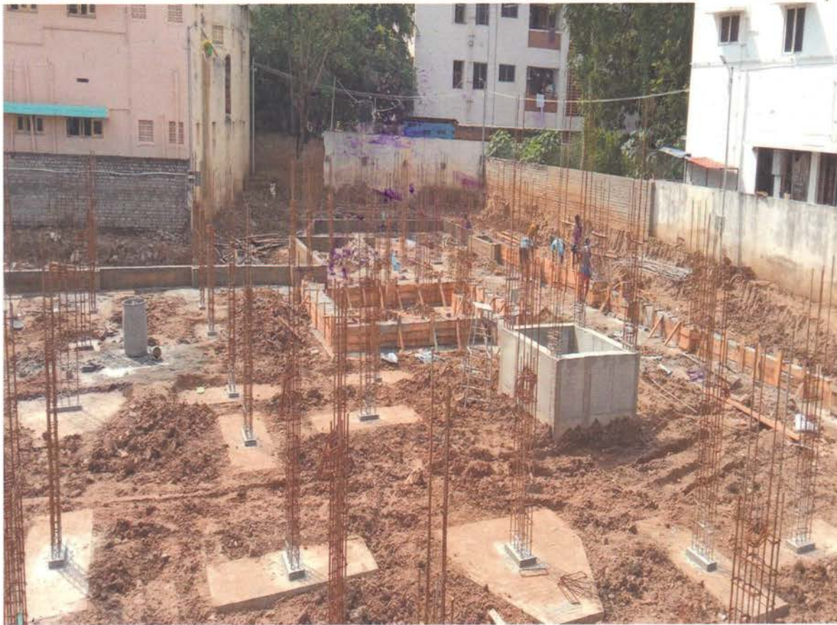
Figure 1 Foundation Completed
