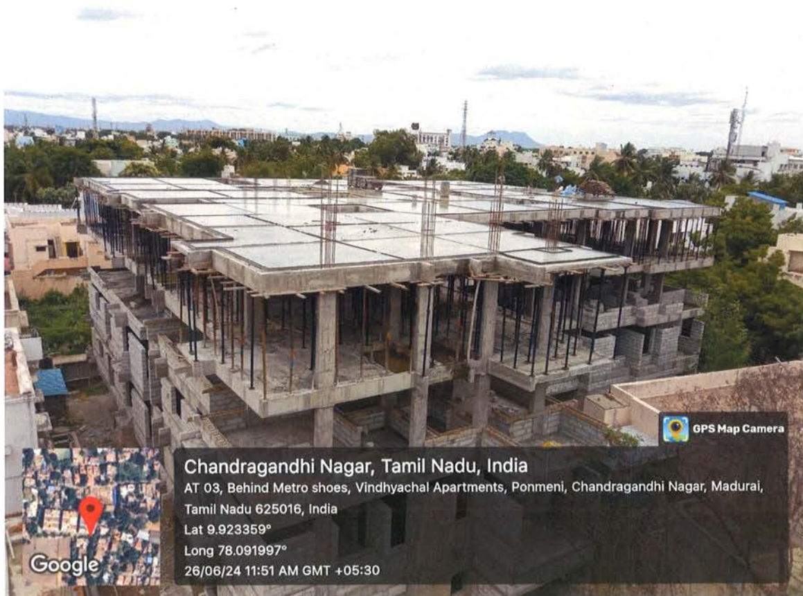
Figure 1 Fourth Floor Roof Completed
