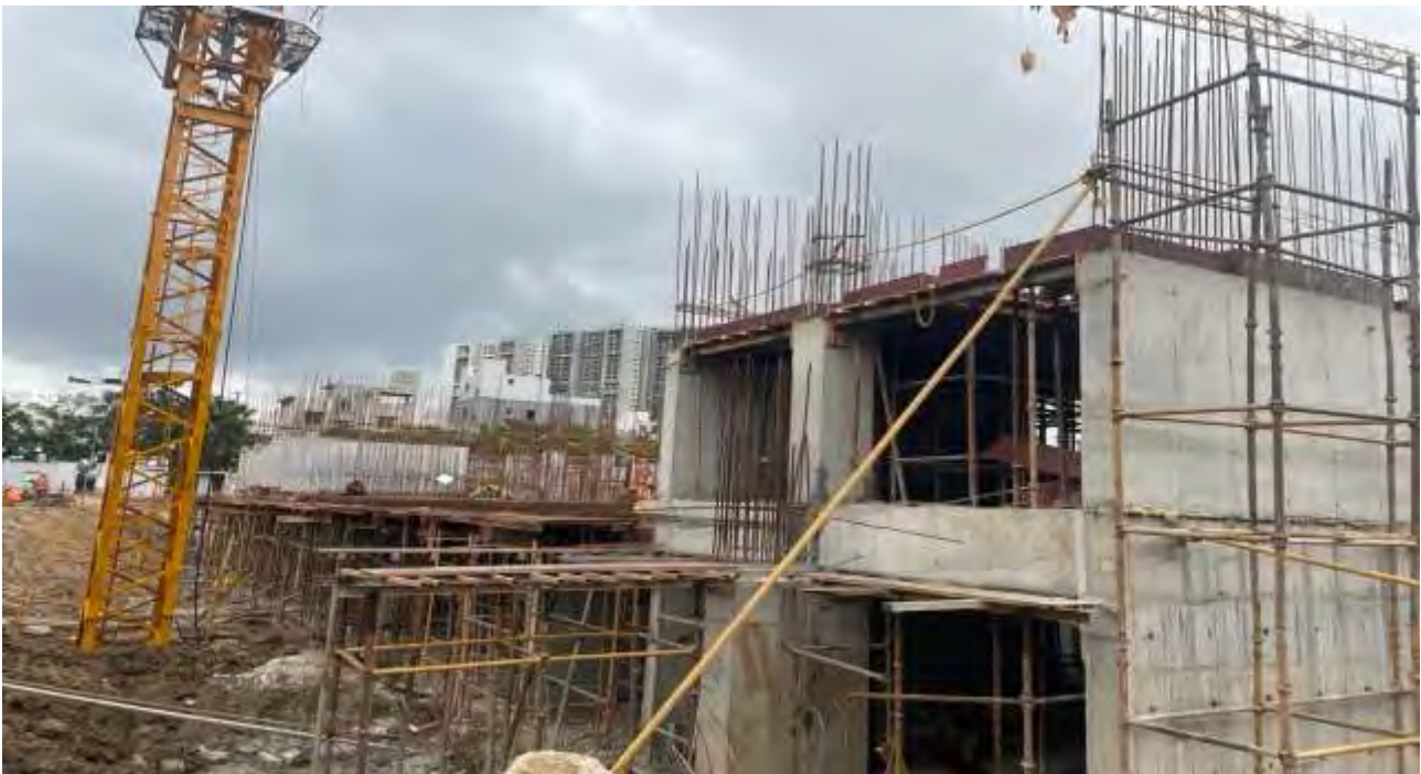
Block A: Stilt Floor and First Floor Slab works in progress.
