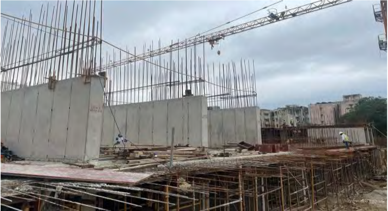
Block A: First Floor Slab works in Progress.
