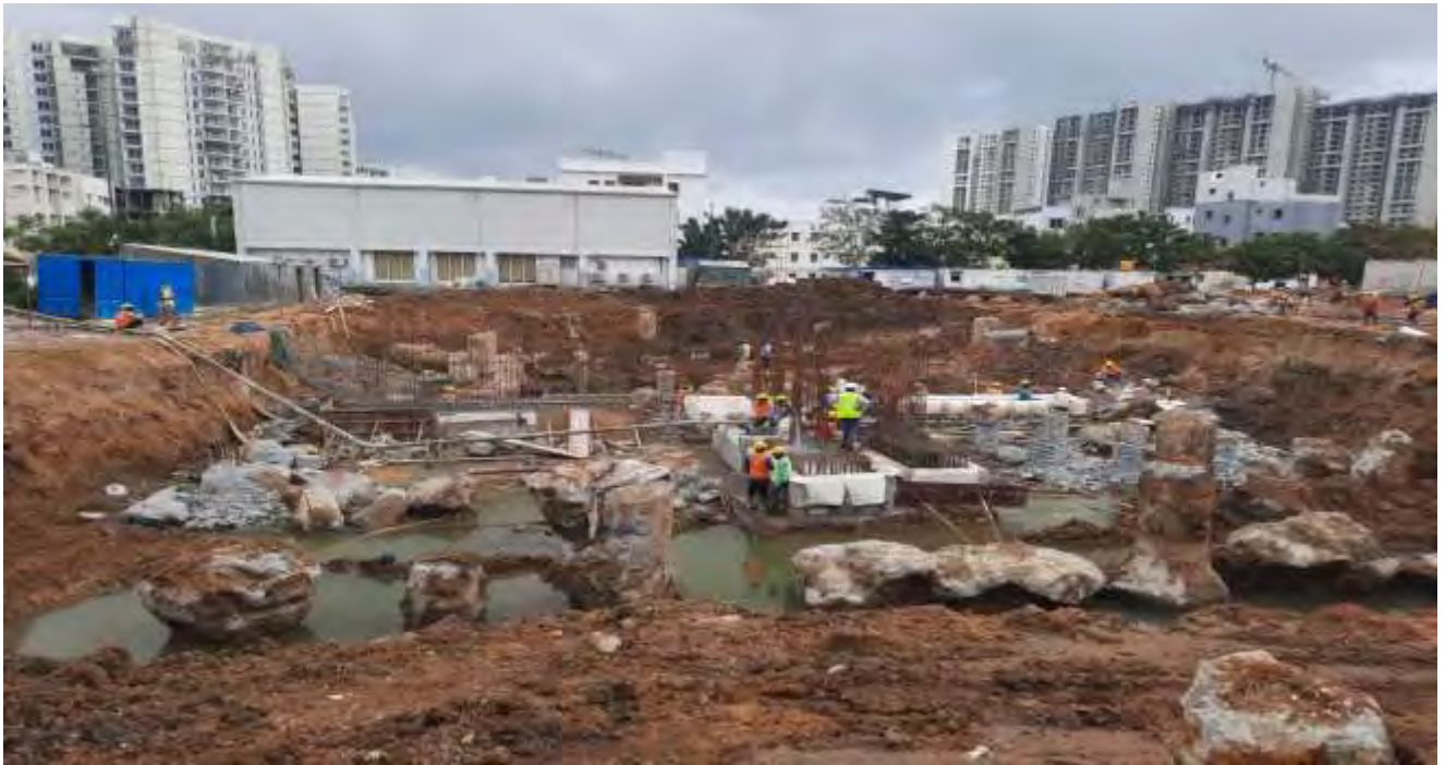
Block B: Pile Works Completed and Foundation in progress.
