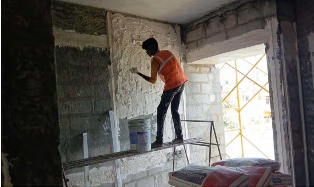
First floor flats gypsum plastering work.
