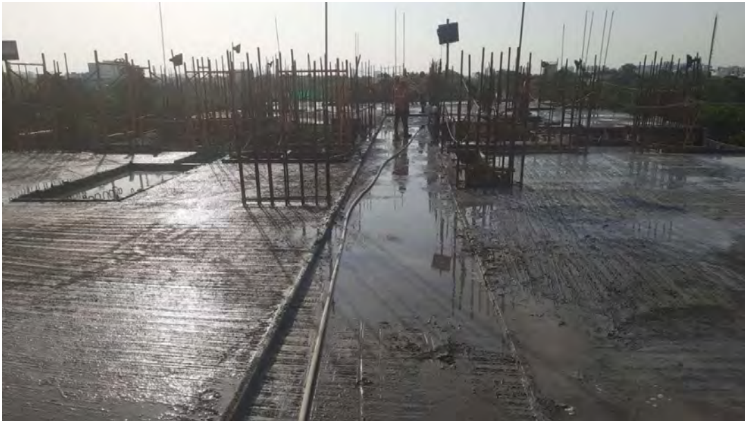
Phase 2 - Fourth floor roof slab concrete work.
