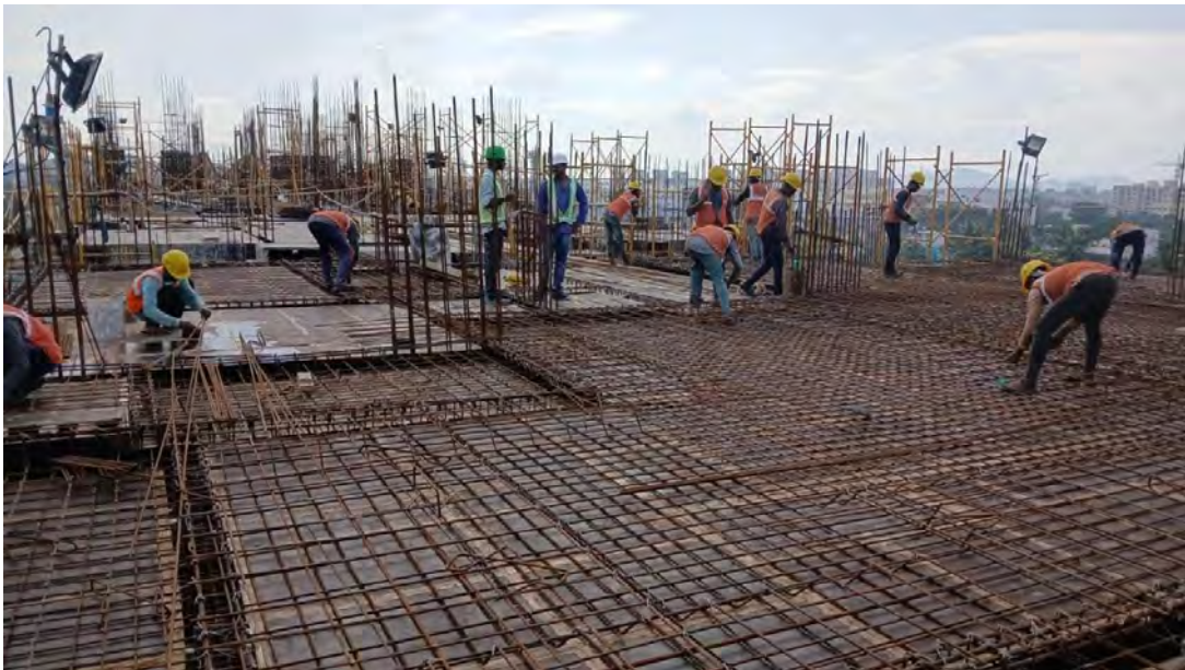
Phase 2 - Fourth floor roof slab reinforcement work.
