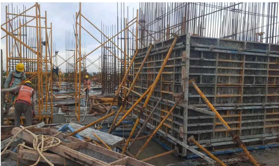
Phase 1 - Fifth floor column and Lift wall shuttering work.
