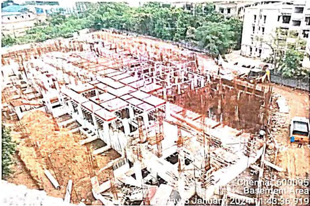
Basement- From South
