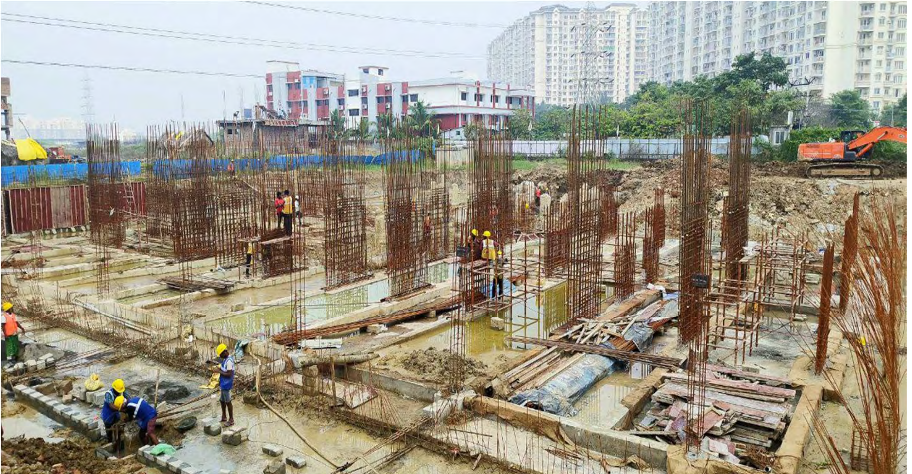
RAFT WORK IN PROGRESS
