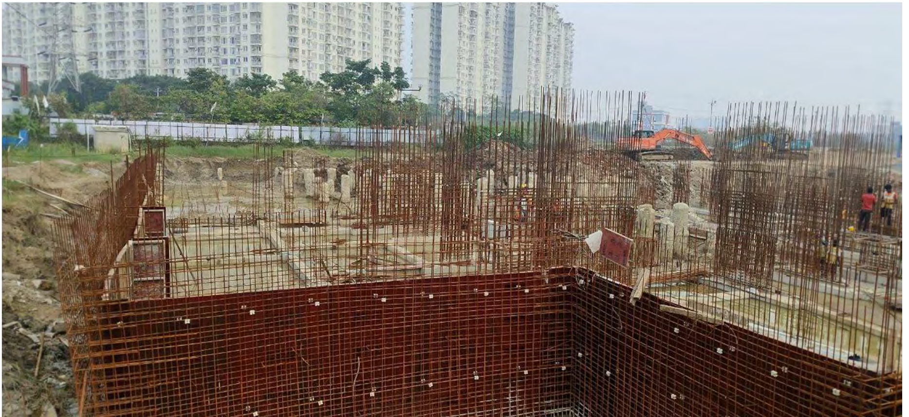
RAFT WORK IN PROGRESS
