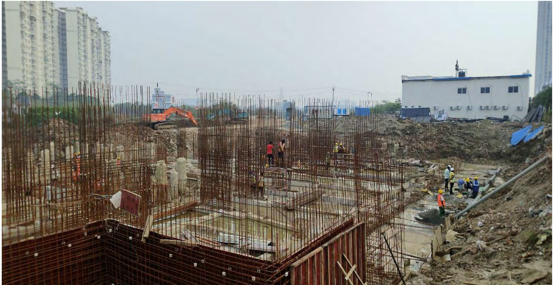
RAFT WORK IN PROGRESS
