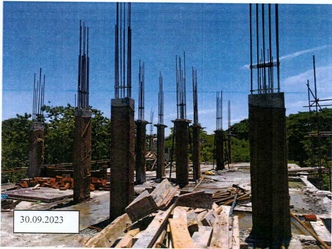
THIRD FLOOR COLUMN CONCRETE WORK IS COMPLETED
