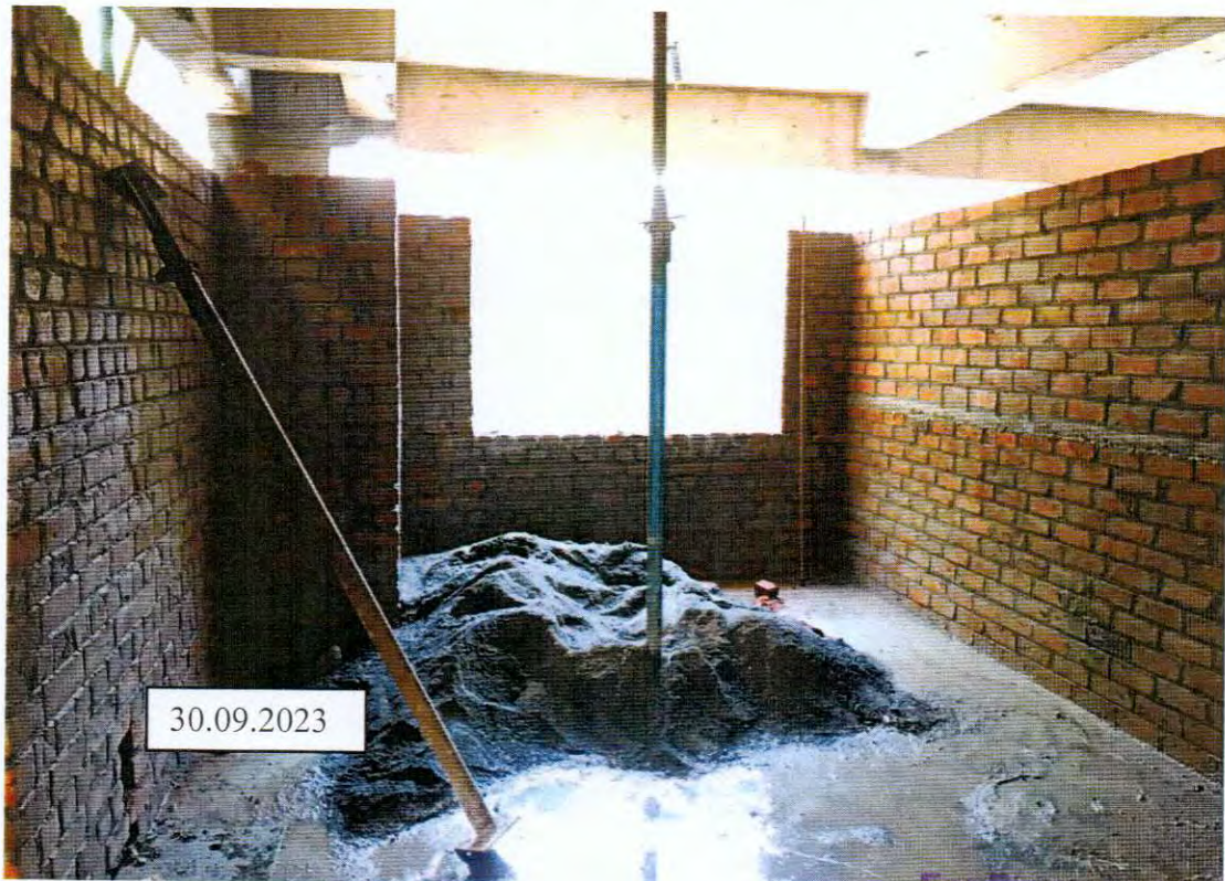
FIRST FLOOR BRICK WORK IS IN PROGRESS
