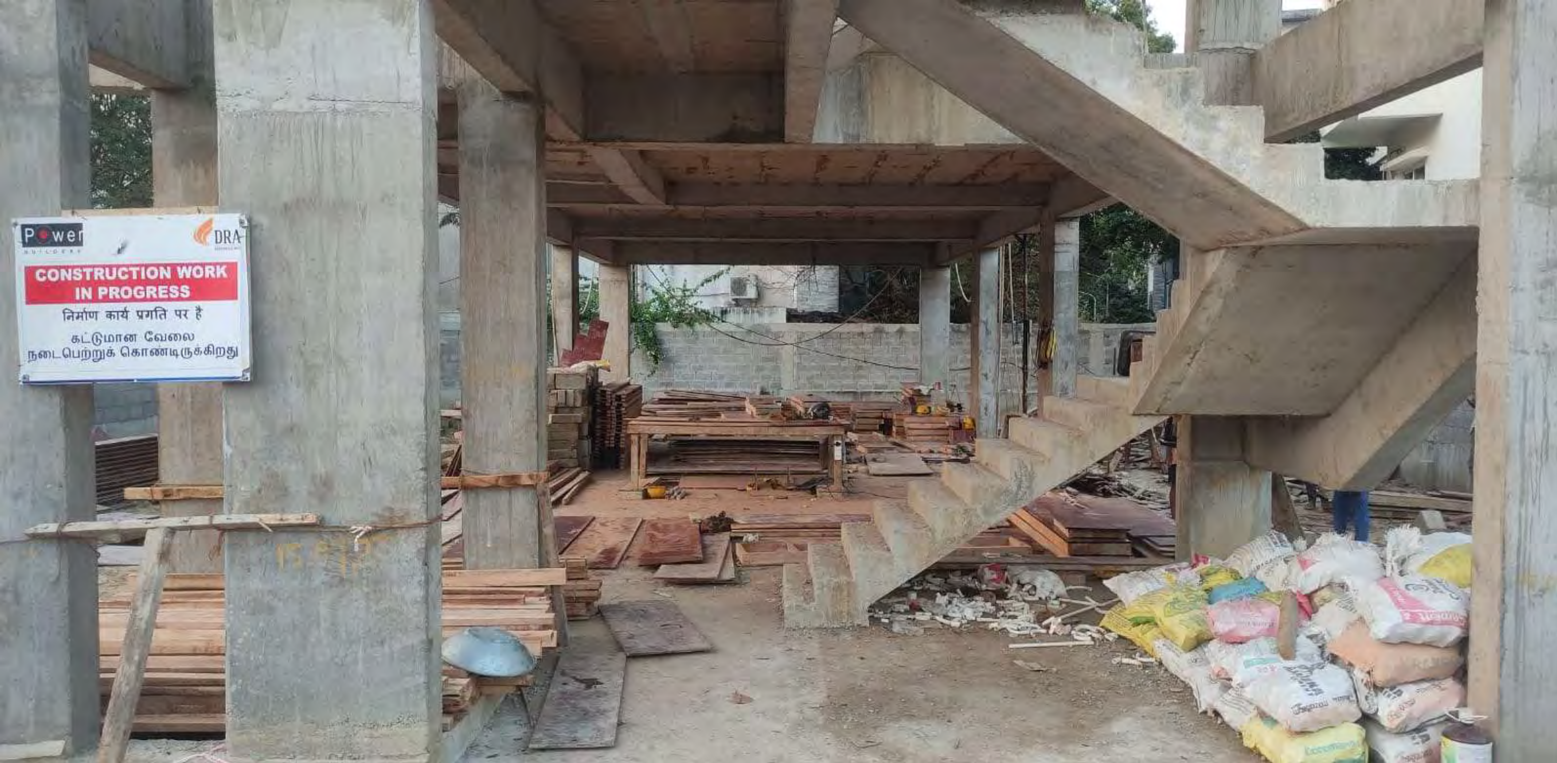
Amenity Block - Grade Slab PCC Work Completed
