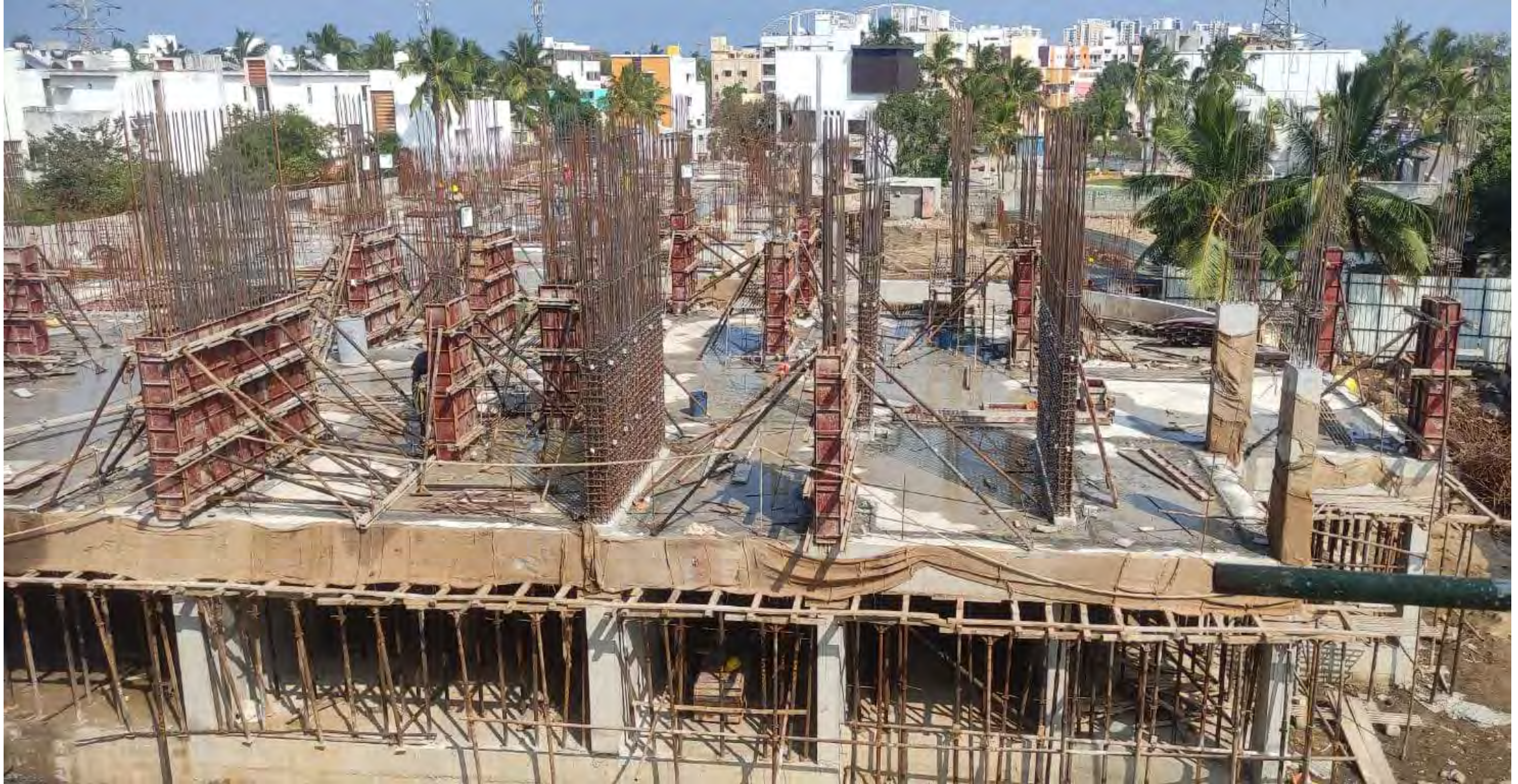
Upper Stilt Floor Column Concreting Work In Progress
