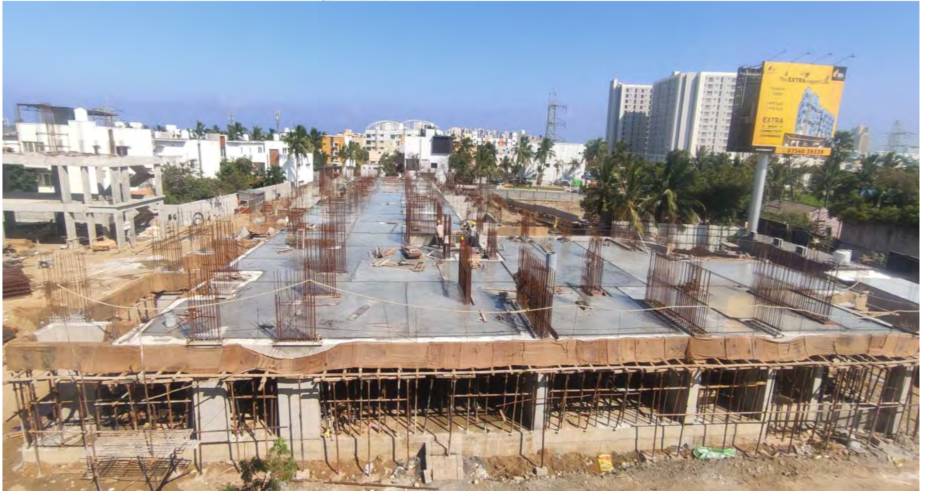
Stilt Floor Roof Slab Work Completed
