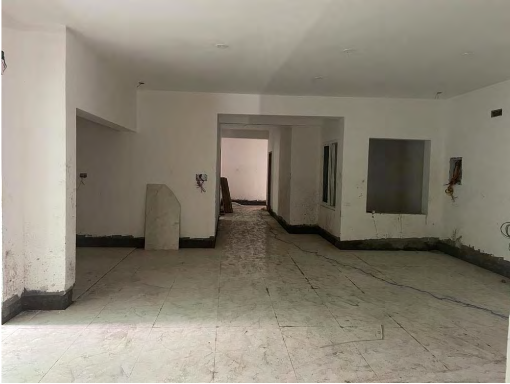
Flooring & Putty Work
