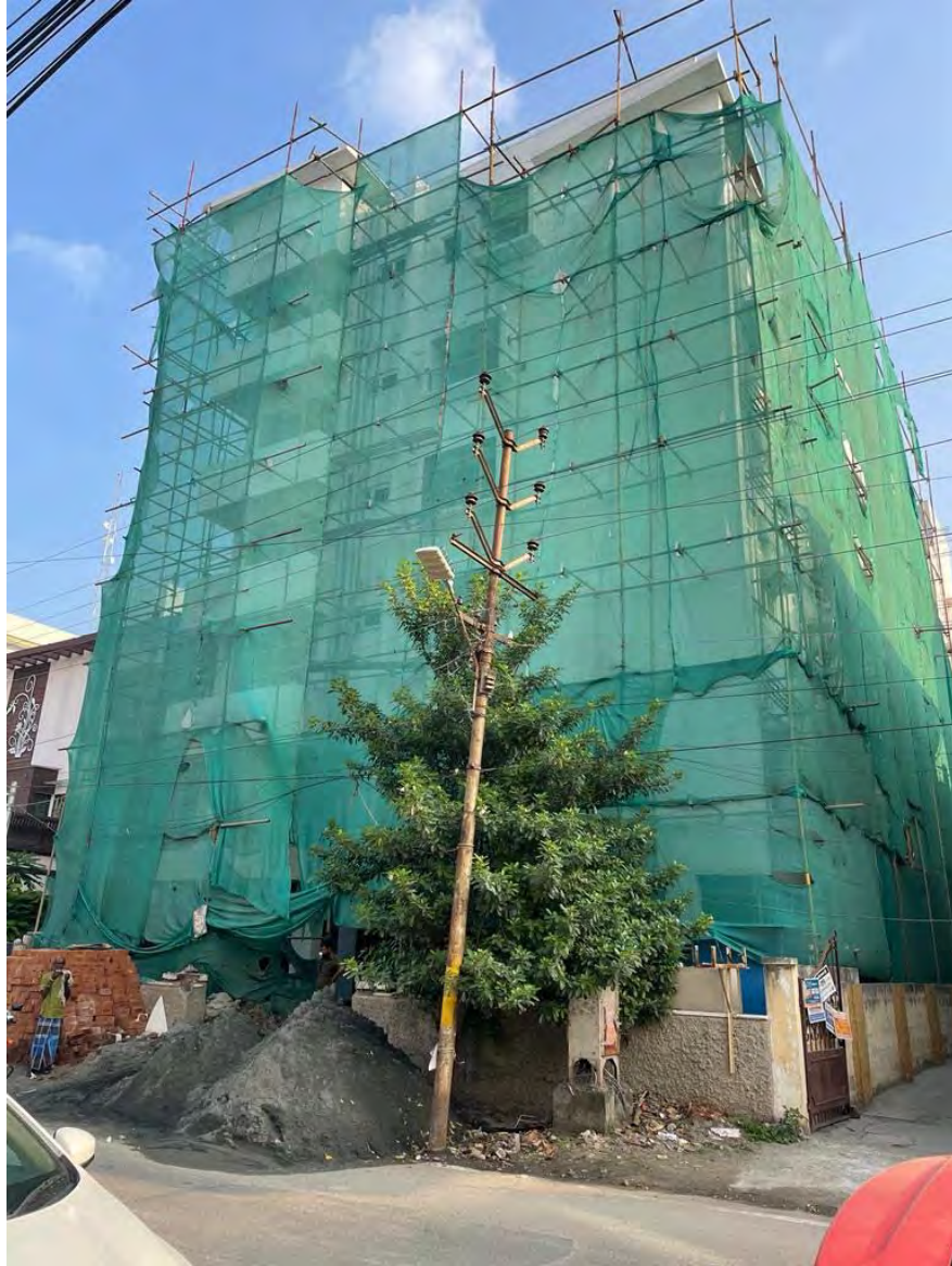
FRONT ELEVATION WORK
