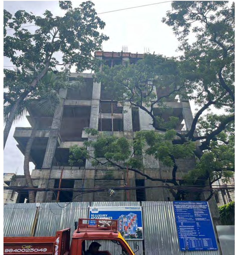
View showing Full building from Chinniah street
