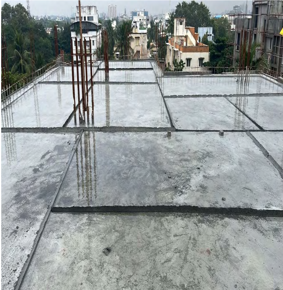
View showing completed Fifth Floor roof concrete
