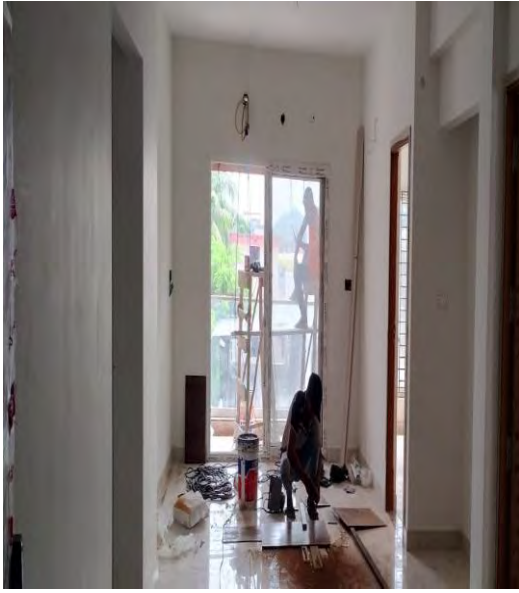
Internal wiring testing work is in progress
