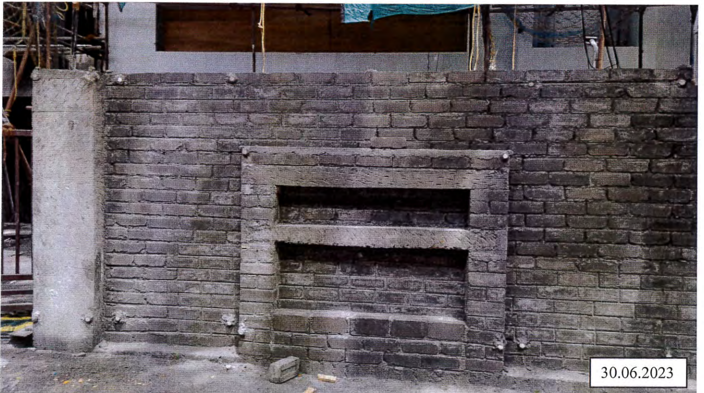
Compound wall work in sin progress (70% completed)
