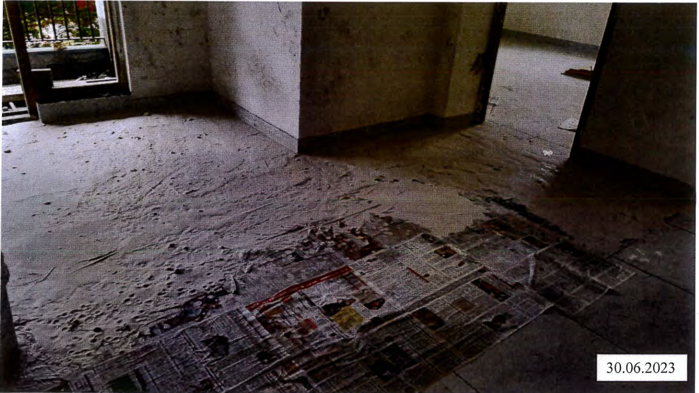
5th floor general flooring work is in progress (90% completed).
