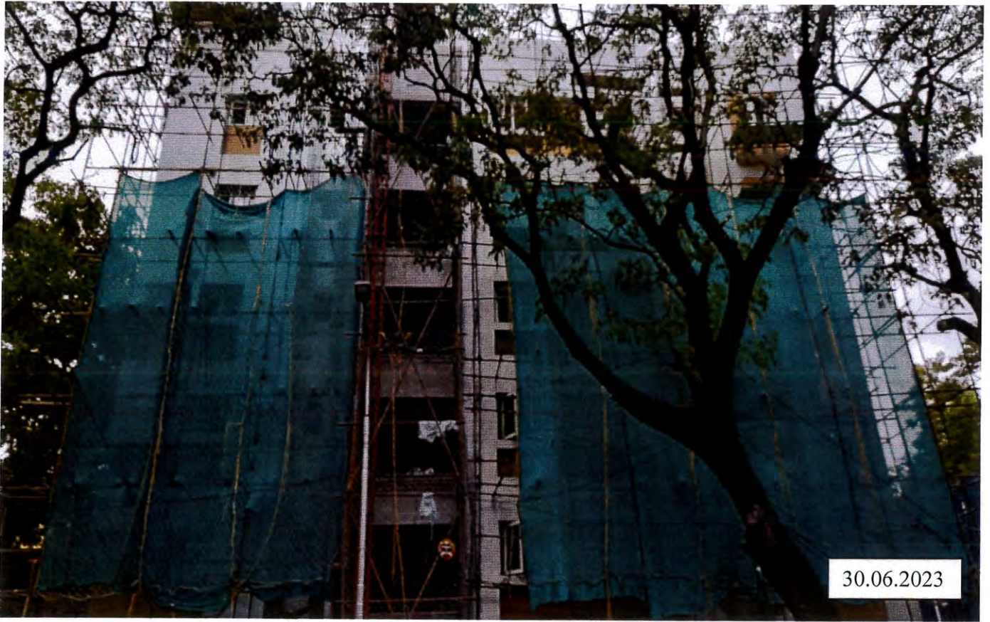
Elevation marble cladding work is in progress
