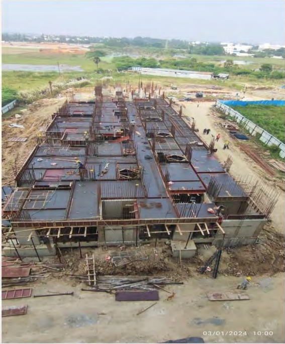
C Block Stilt floor roof Work in progress
