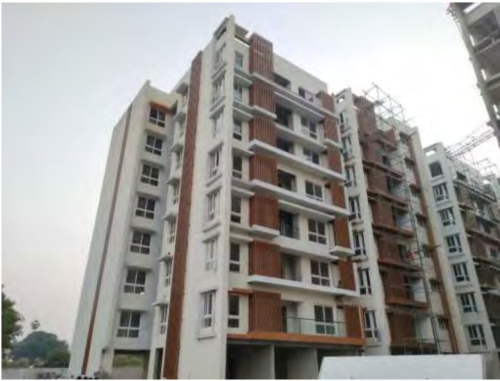
Block 6: Tower J -External Painting & Balcony Railing work in progress
