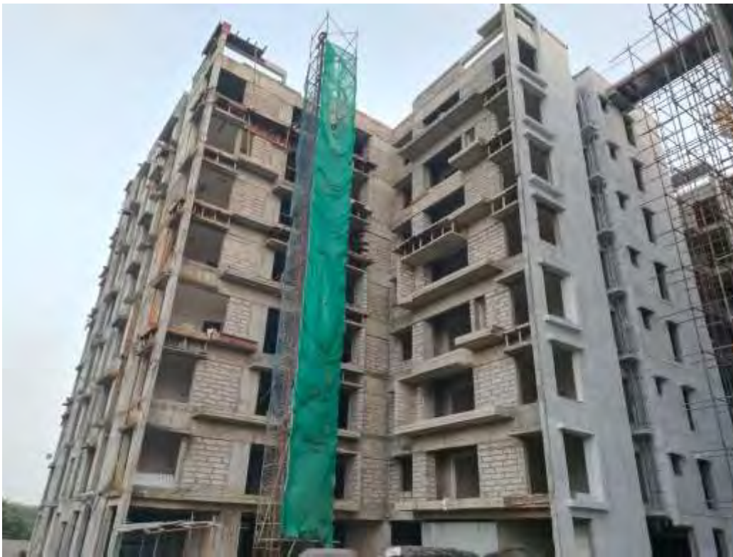
Block 4: External Plastering work in progress.
