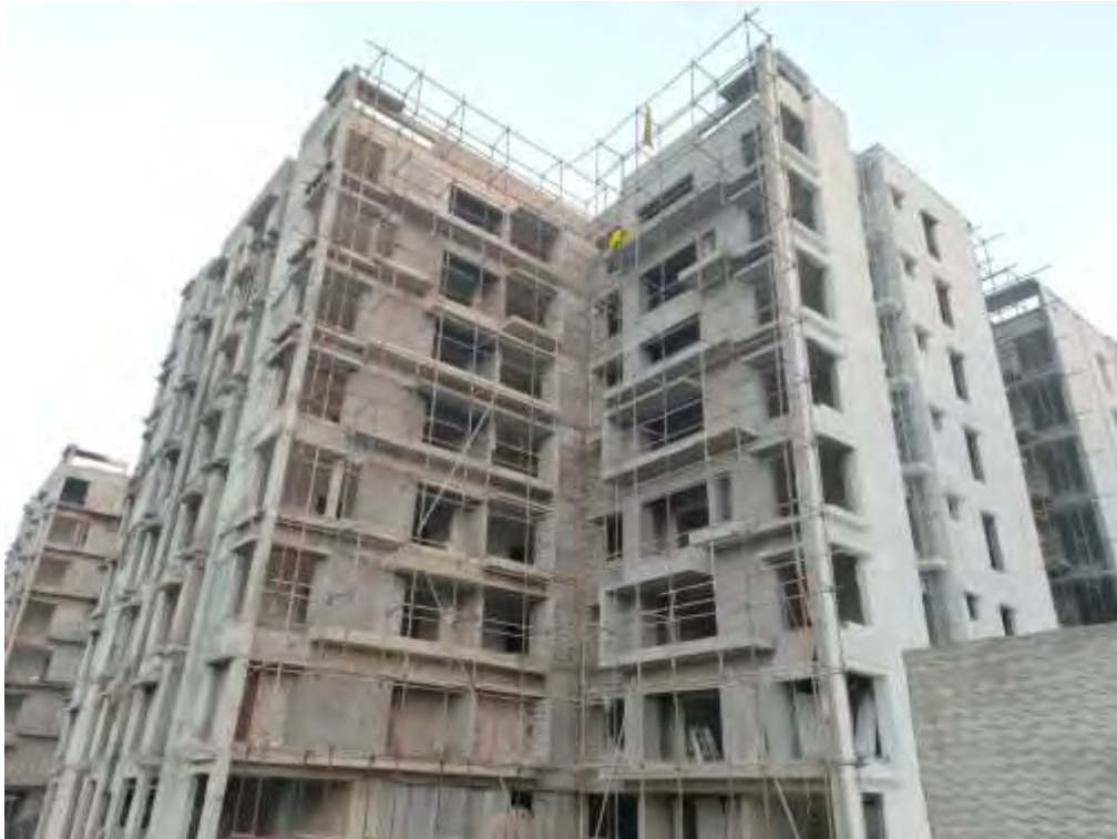
Block 4: External Plastering work in progress.
