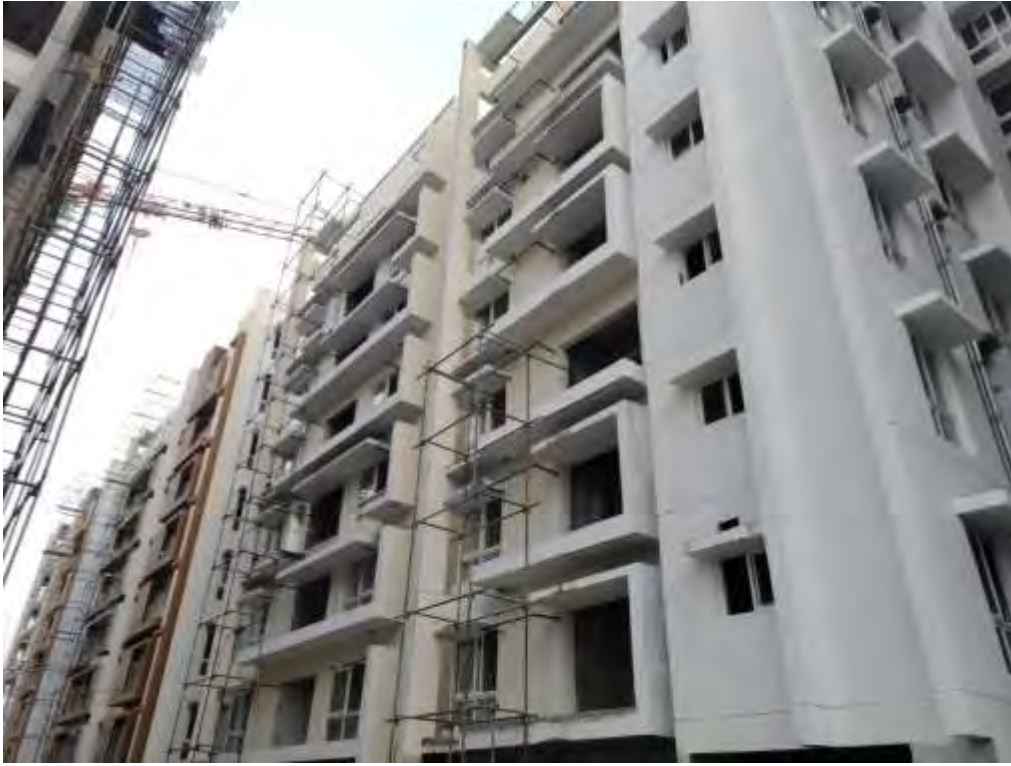
Block 6 : Tower H – External Painting work in progress
