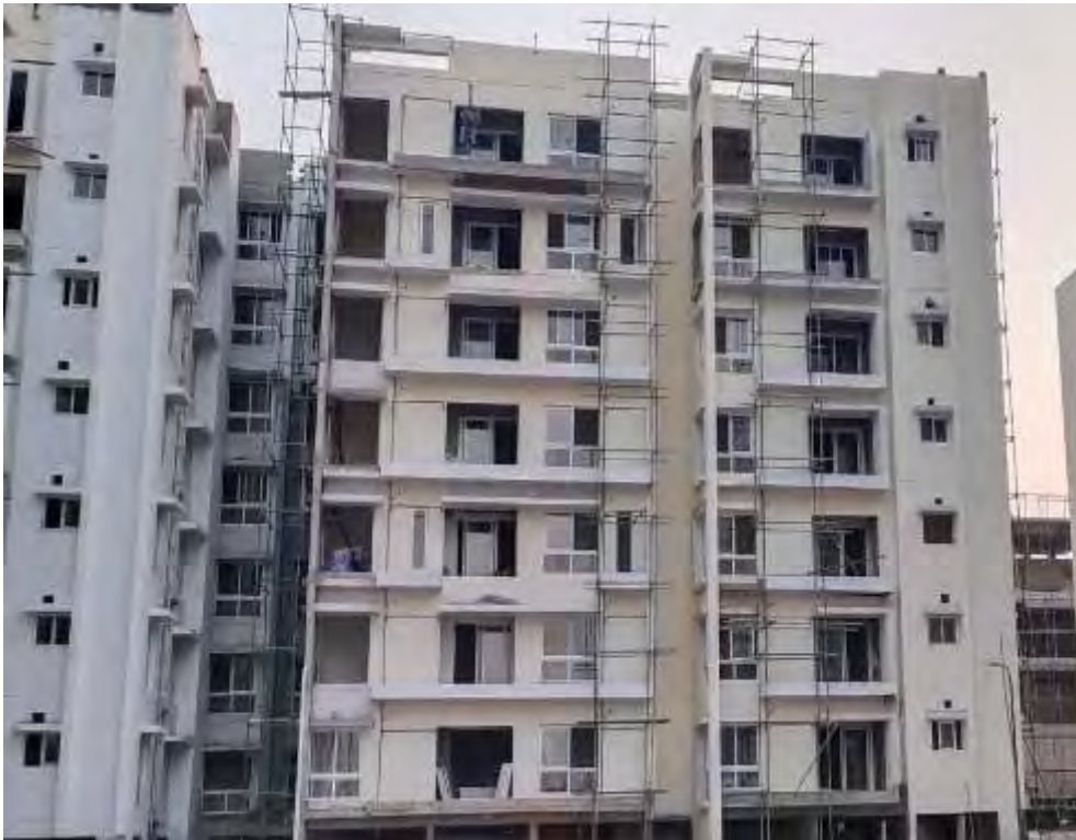
Block 6 : Tower G – External Painting work in progress
