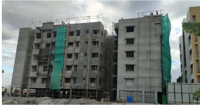
BLOCK - C - CURING WORK
