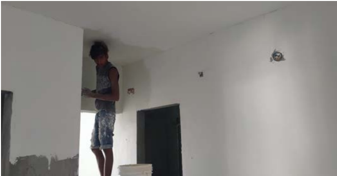
BLOCK - C - INTERNAL PLASTERING WORK
