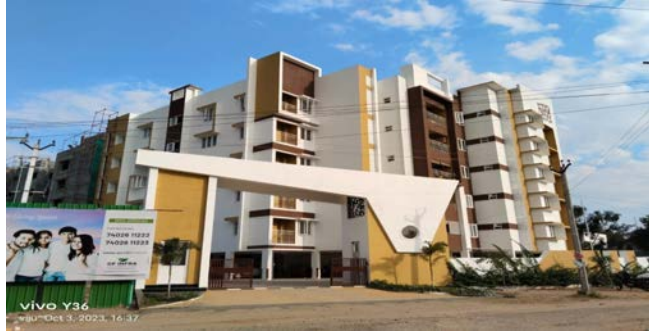
BLOCK - C - EXTERNAL WALL PLASTERING WORK
