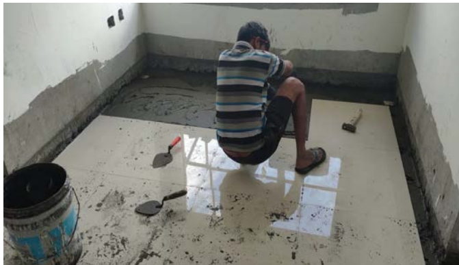
BLOCK - C - FLOORING TILES LAYING WORK
