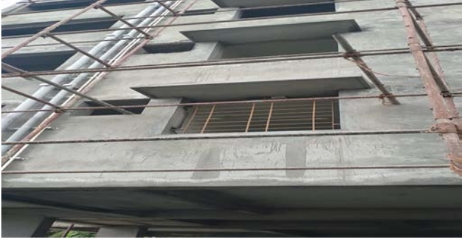
BLOCK - C - INTERNAL PAINTING WORK
