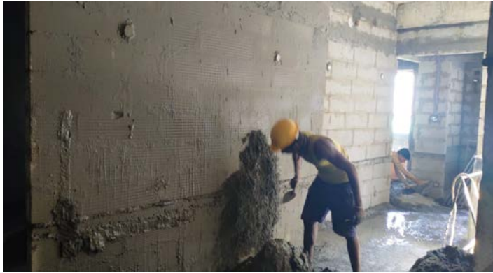
BLOCK - C - TOILET SUNKEN WATER PROOFING WORK
