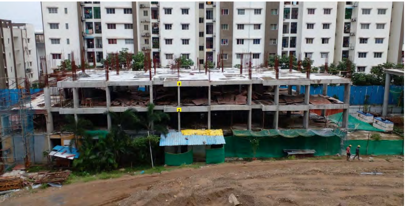
BLOCK D – THIRD FLOOR PART SLAB CONCRETE WORK
