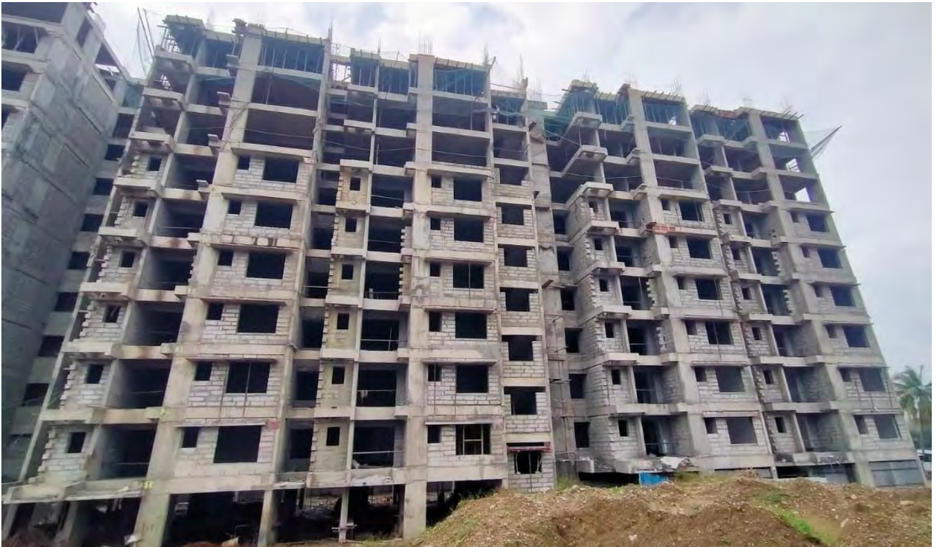
BLOCK A – TENTH FLOOR PART SLAB CONCRETE WORK
