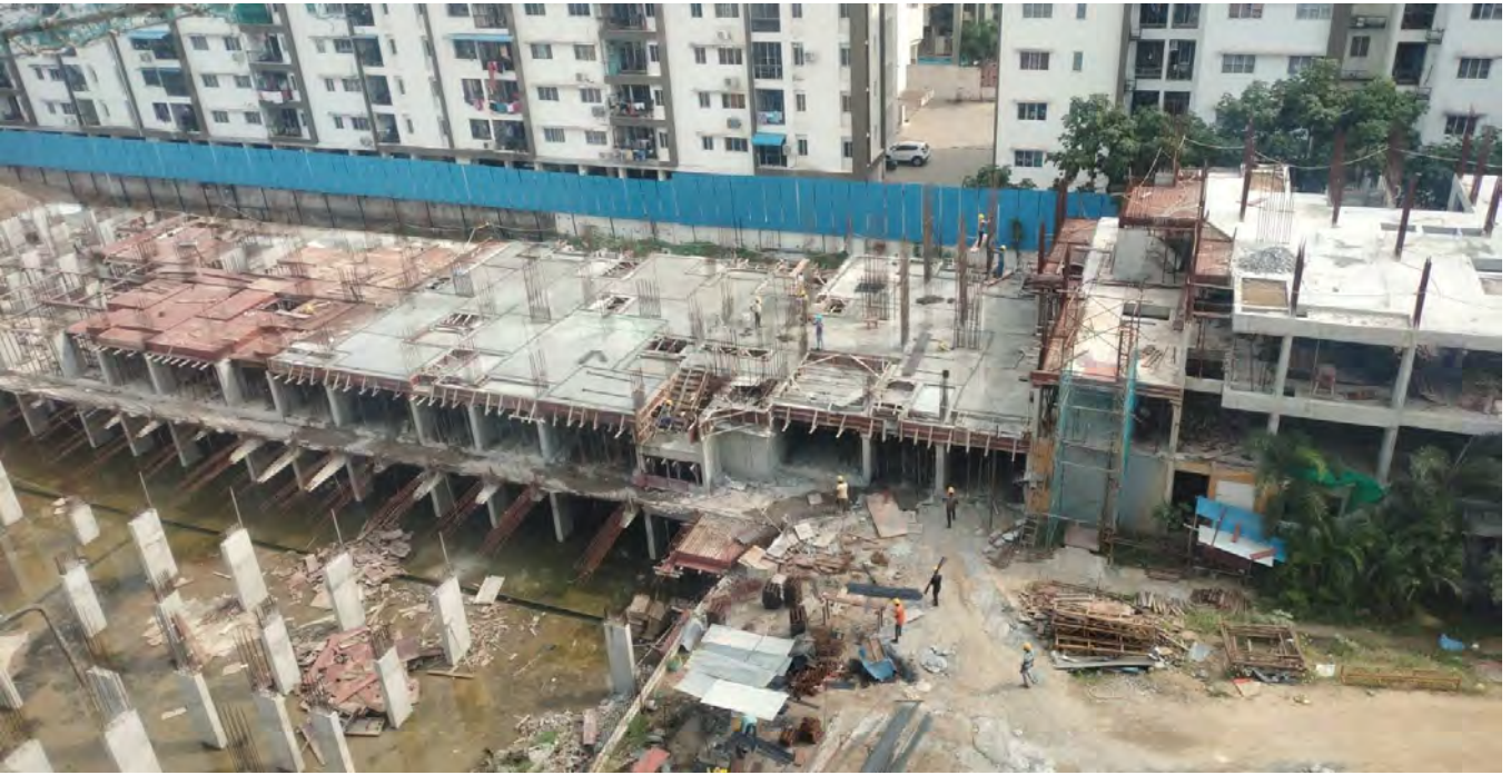
BLOCK D – FIRST FLOOR PART SLAB CONCRETE WORK
