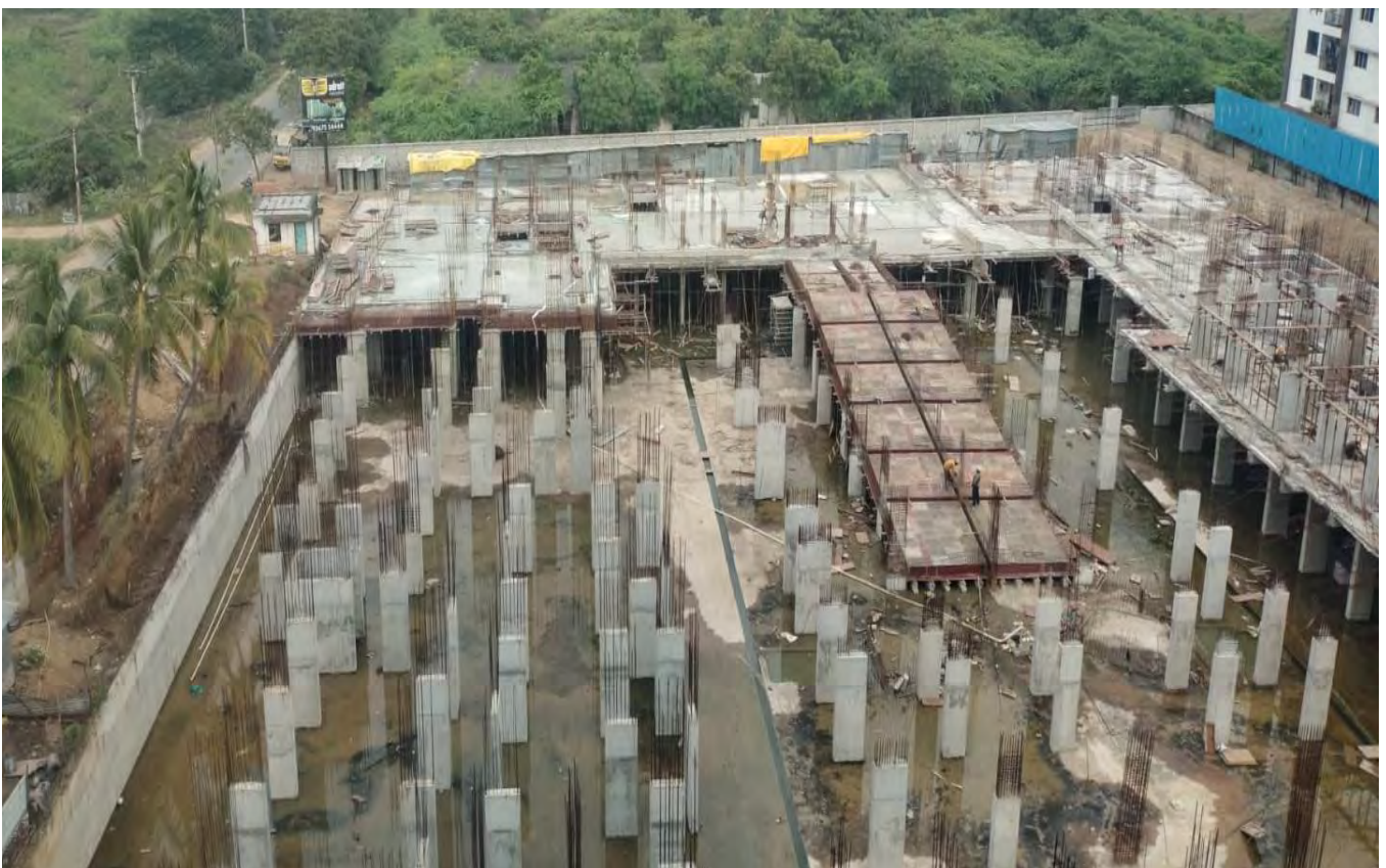
BASEMENT – BLOCK B BASEMENT ROOF SLAB PART AREA CONCRETE WORK
