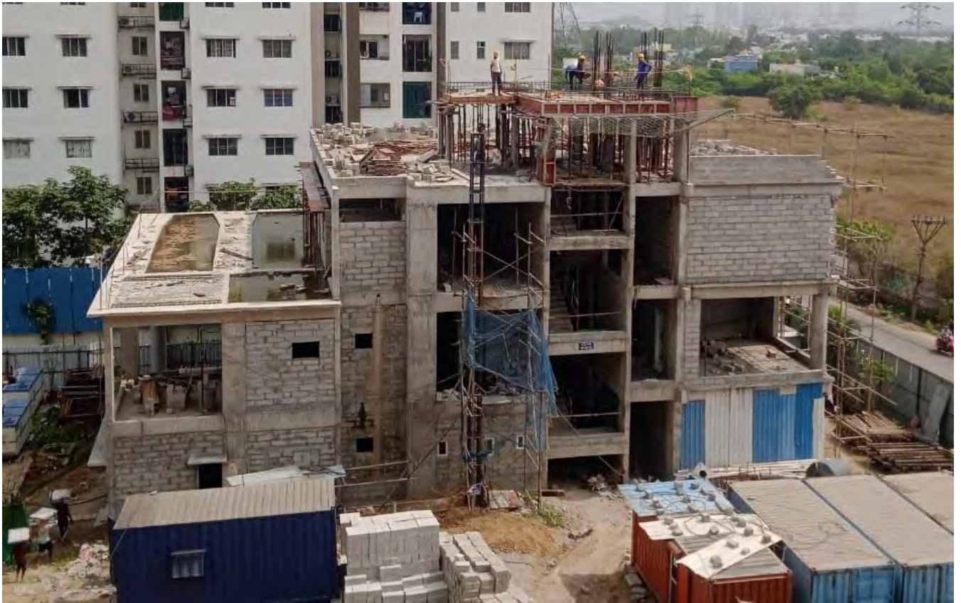
CLUB HOUSE – WEST SIDE VIEW
