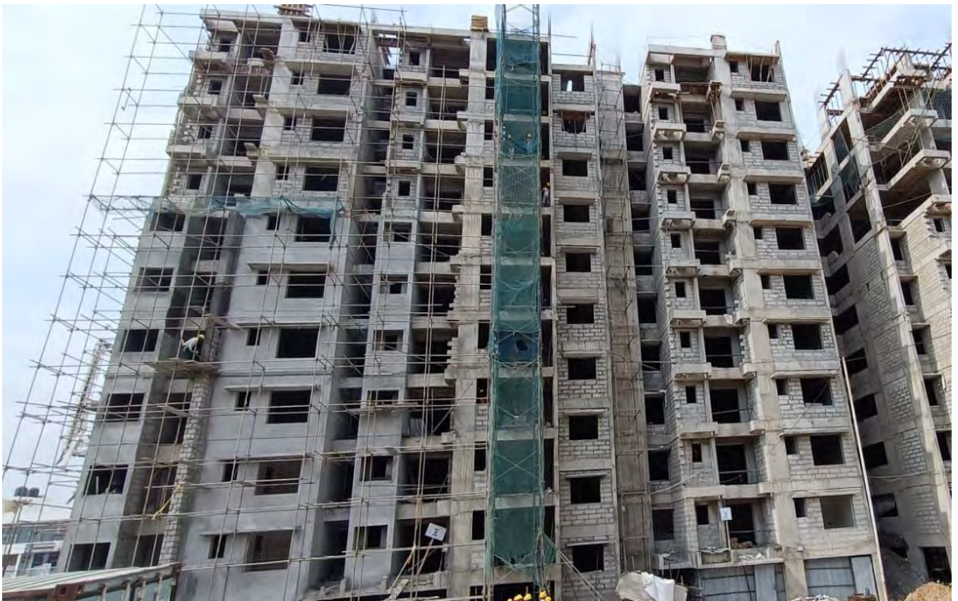
BLOCK A – TERRACE FLOOR PART SLAB CONCRETE WORK
