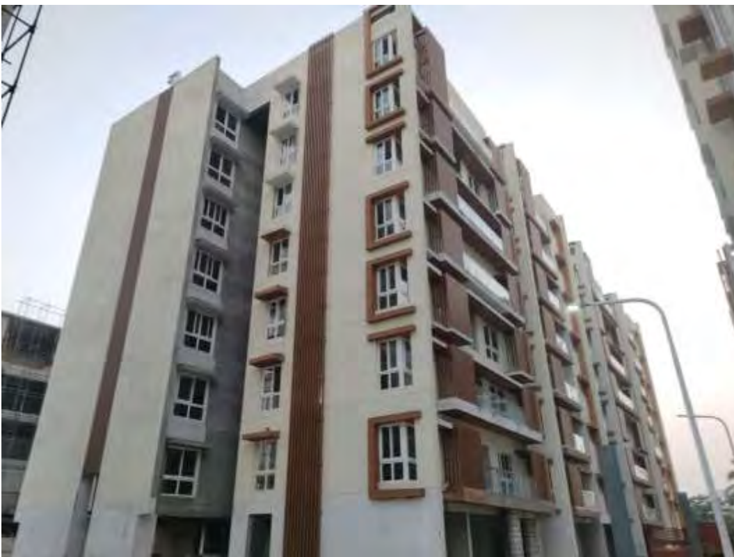
Block 5: Tower F – External Painting, Balcony Railing in Progress.
