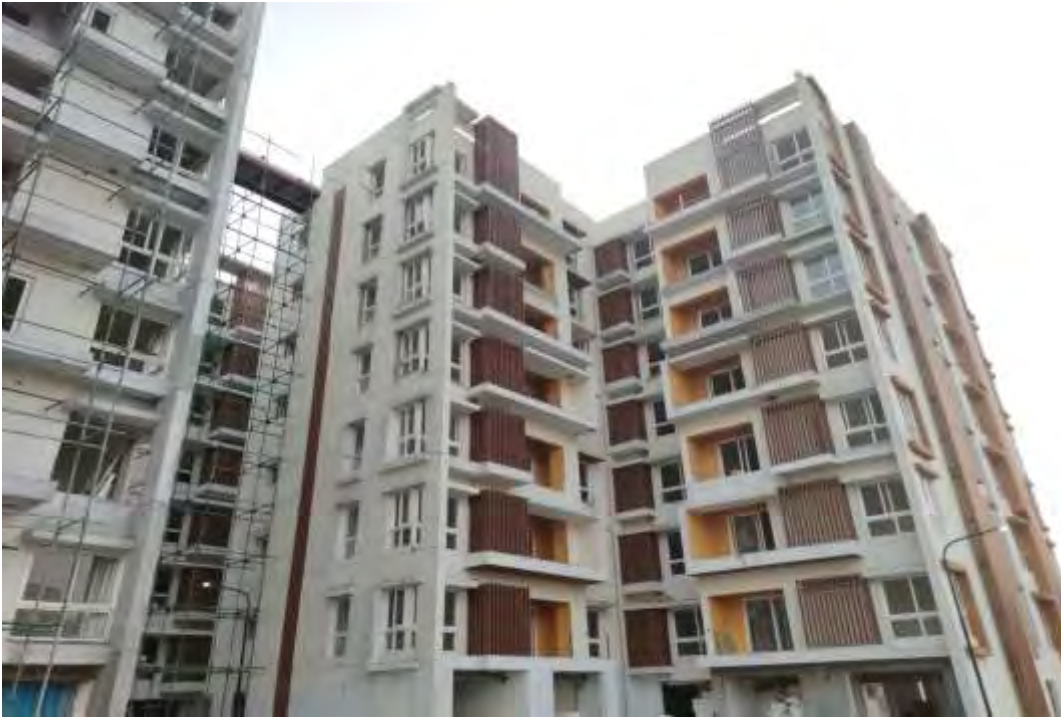
Block 1: External painting and Balcony Railing work in progress
