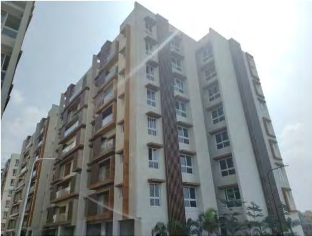
Block 5: Tower E –External Painting work in Progress
