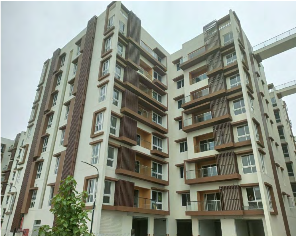
Block 2: External Painting & Common area painting works in progress
