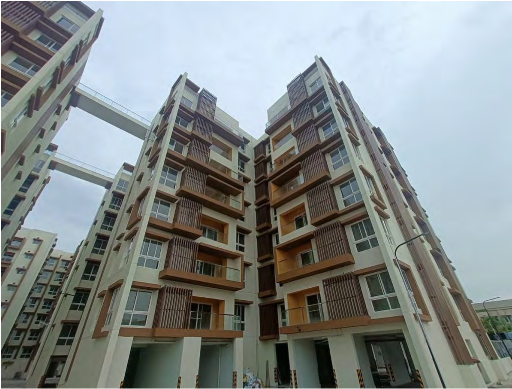
Block 1: External painting and Common area Painting in progress
