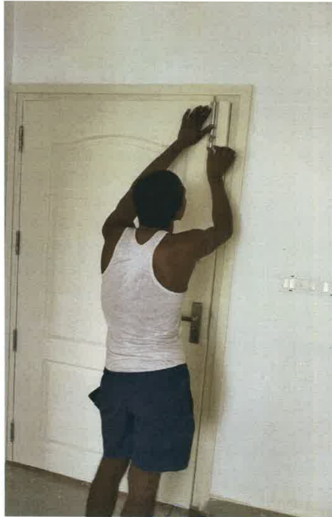
BLOCK 8 – TOWE BOLT FIXING WORK
