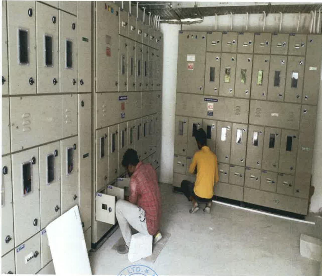
BLOCK – 8 EB ROOM METER PANEL FIXING WORK
