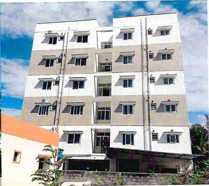
Photo taken on 15.09.2022 – North side view
