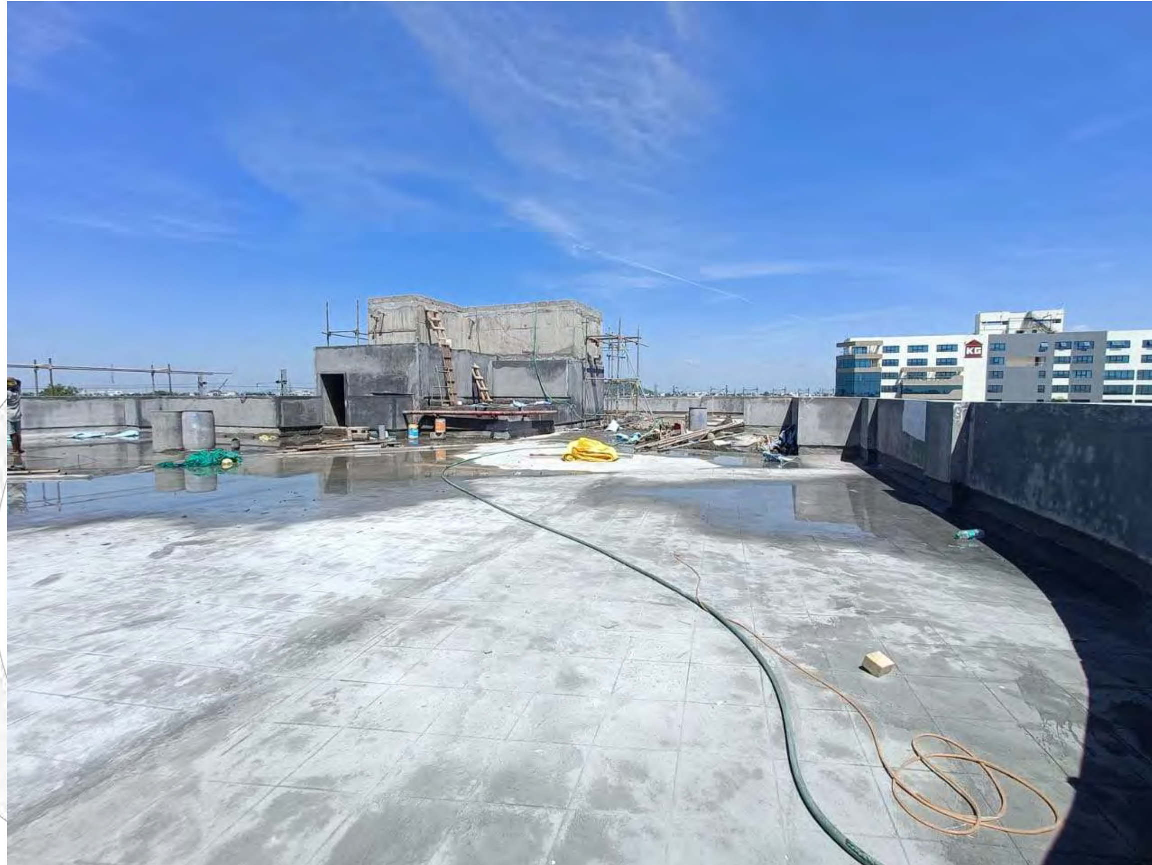
Terrace Waterproofing Work Completed
