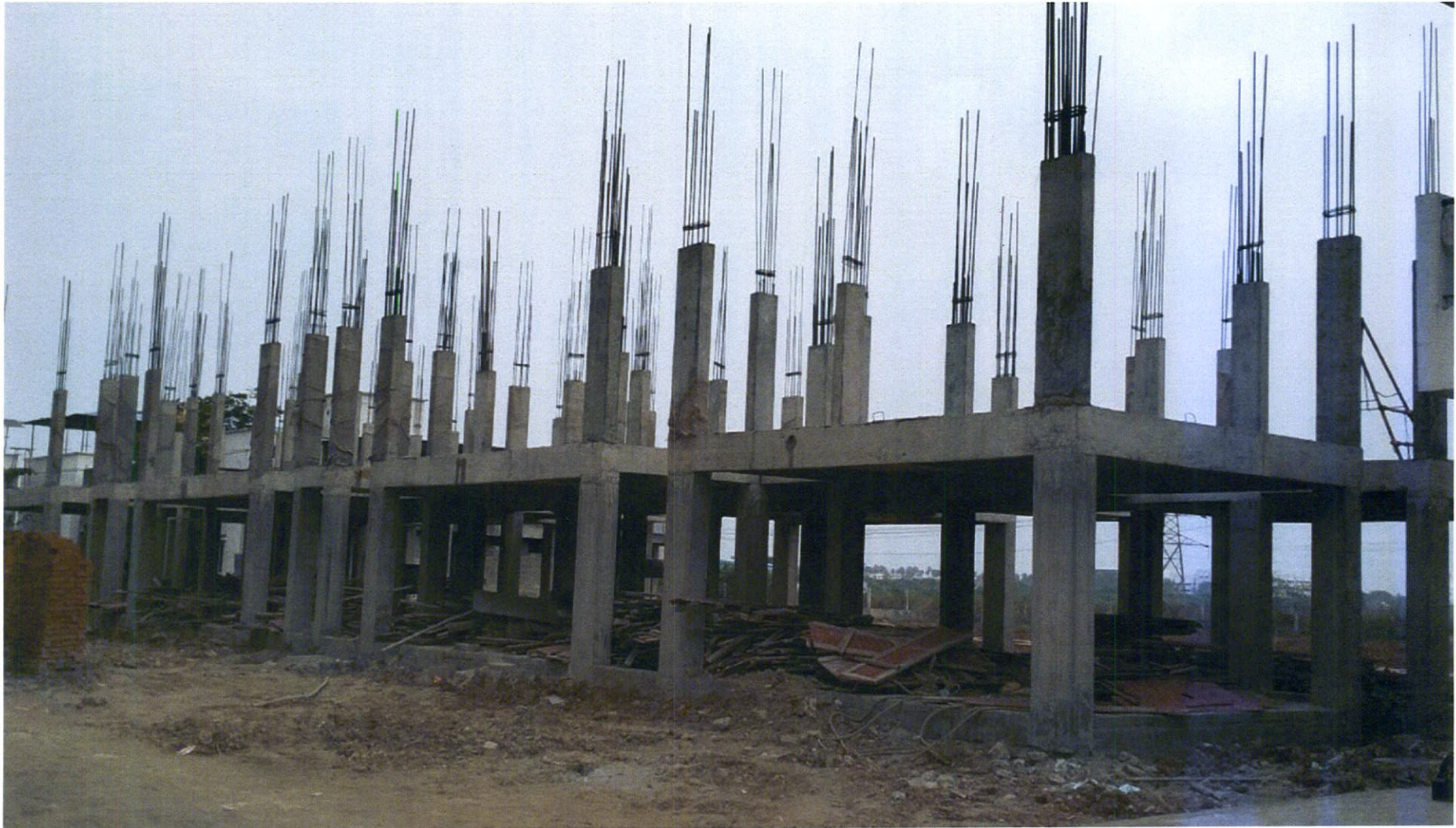
BLOCK-10 STILT 1ST ROOF COLUMN COMPLETED
