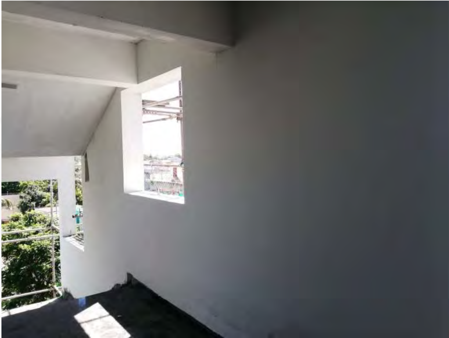
Lobby Painting Work In Progress
