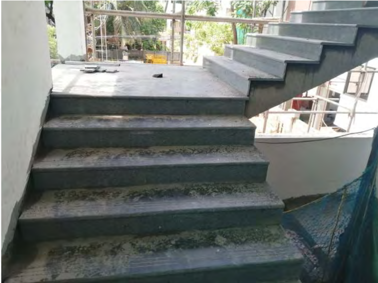
Staircase Granite Work In progress
