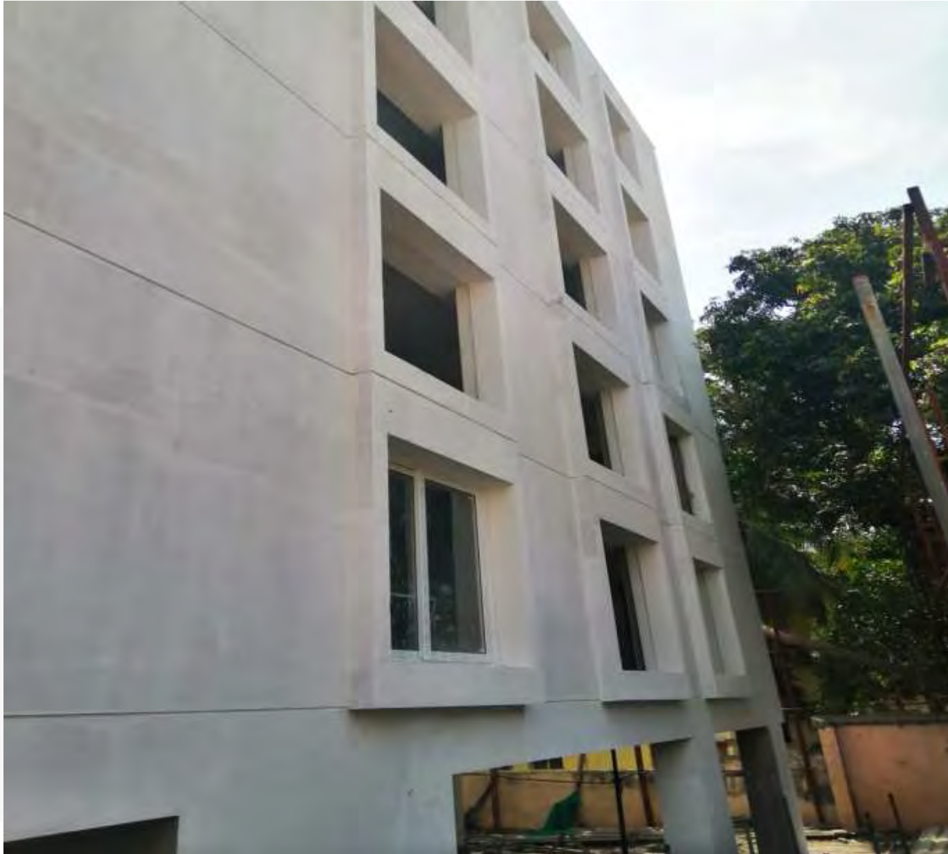
External Painting Work in Progress
