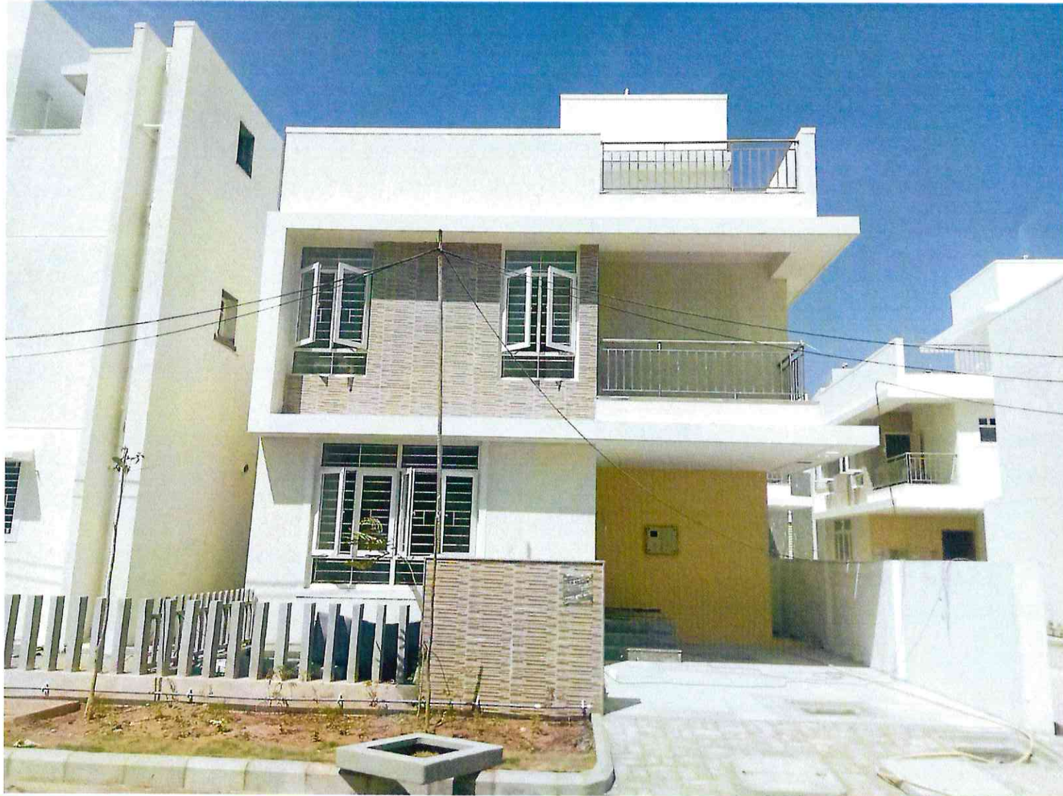
Plot No. 7A - Flooring & Painting work completed
