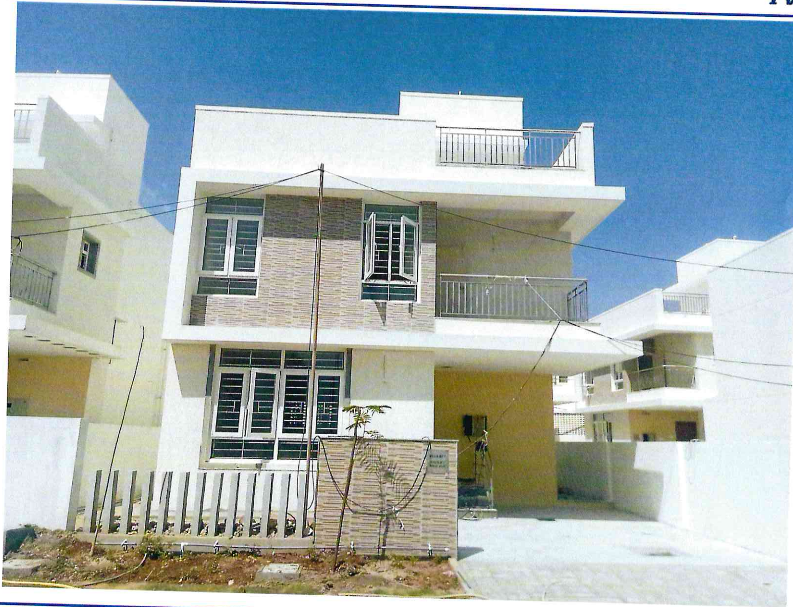
Plot No.8A – Flooring & Painting work completed
