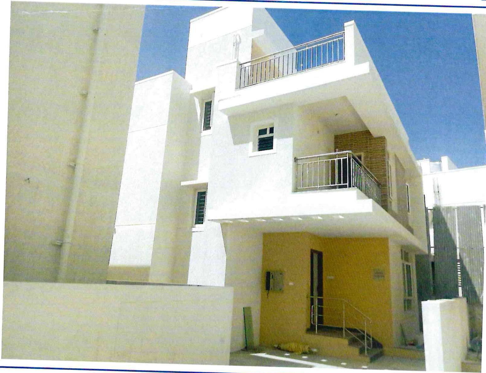
Plot No. 7B – Flooring & Painting Completed
