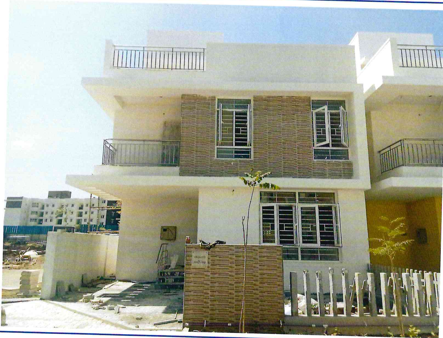
Plot No.1C - Flooring & Painting work Completed
