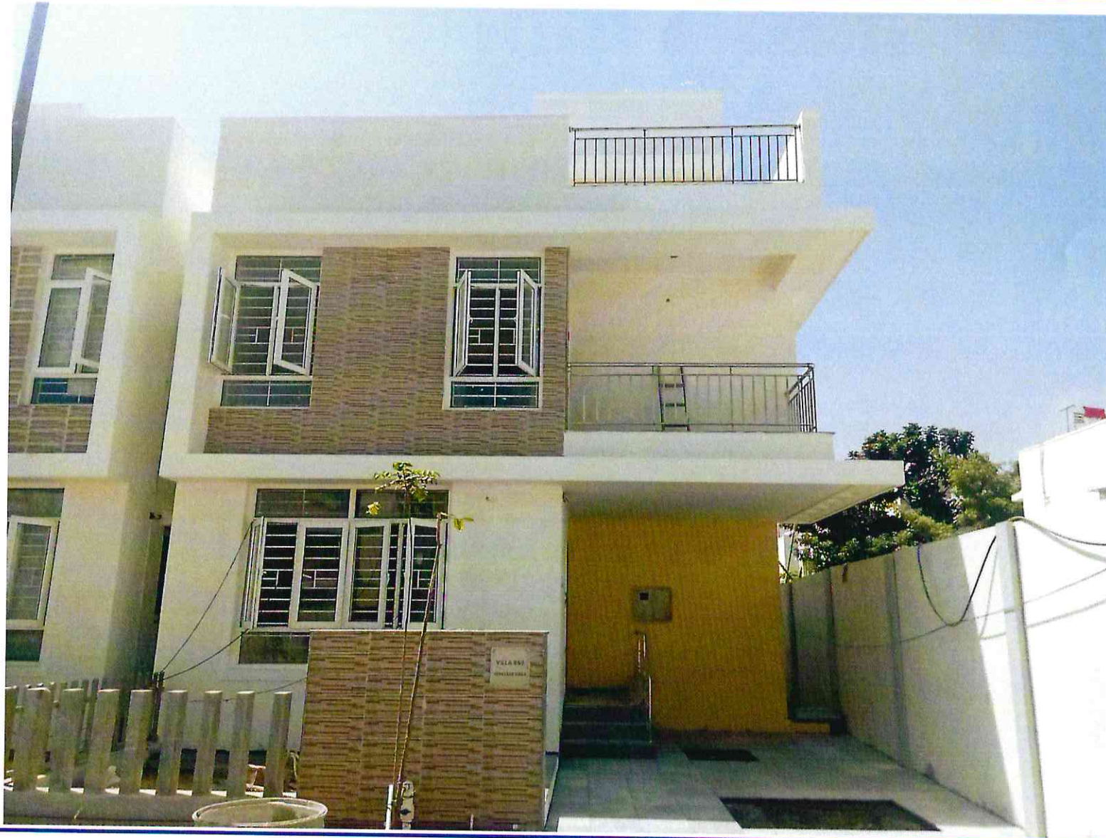
Plot No.1A - Flooring & painting work completed
