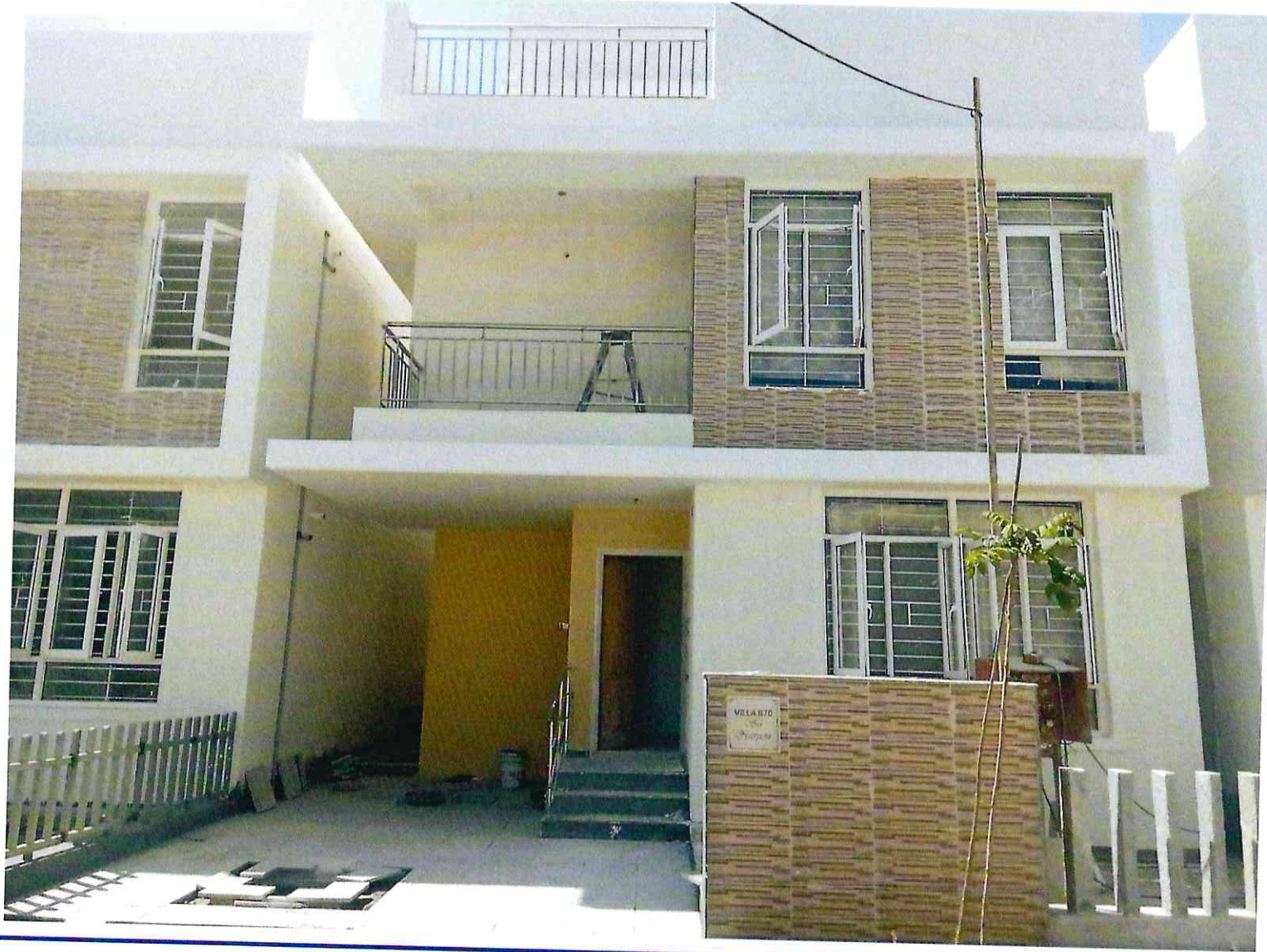
Plot No.1B - Flooring & Painting work completed
