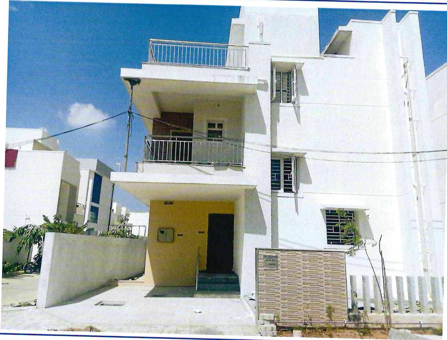
Plot No.06 – Flooring & Painting work completed
