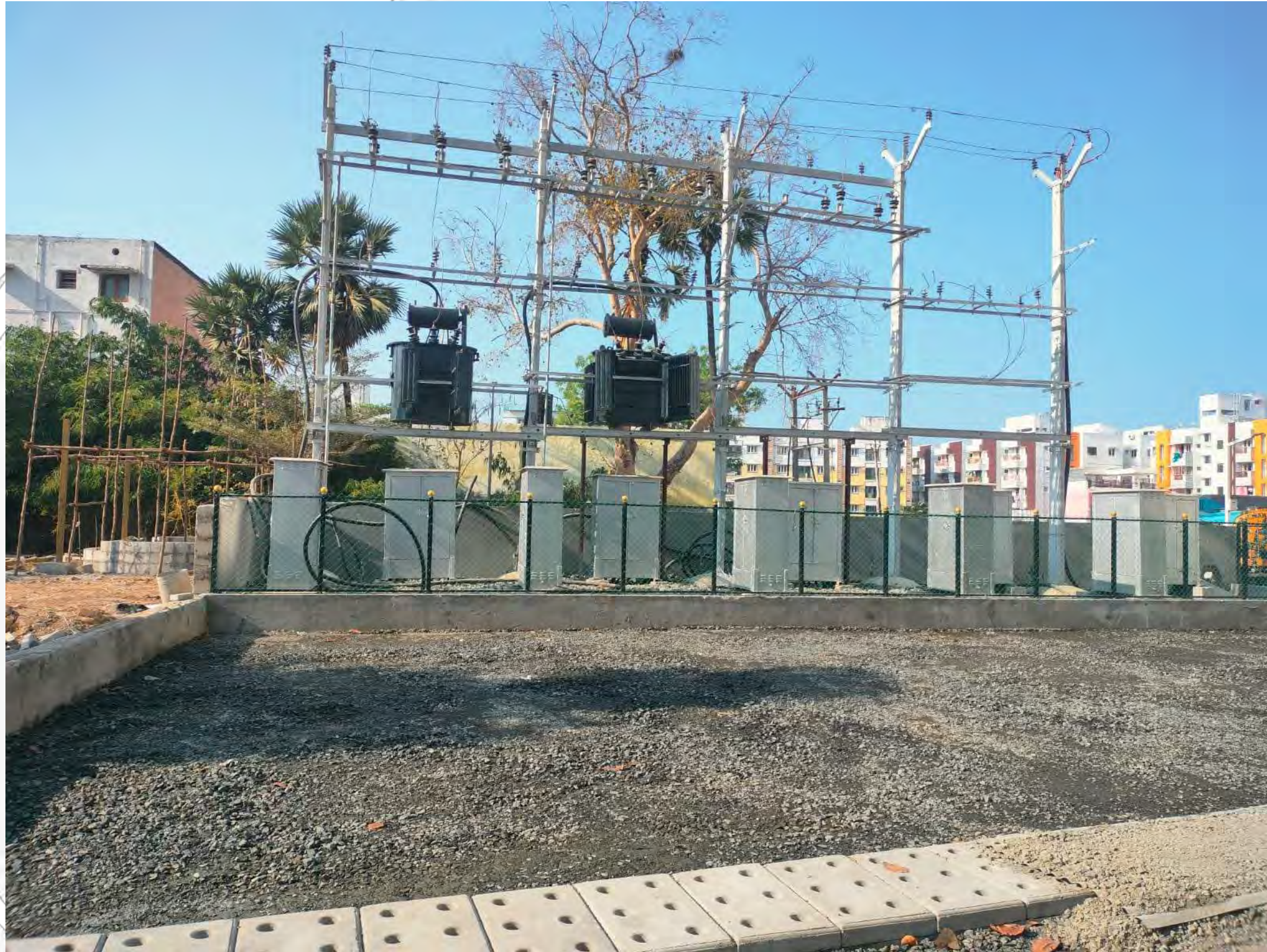
Transformer Yard Work Completed
