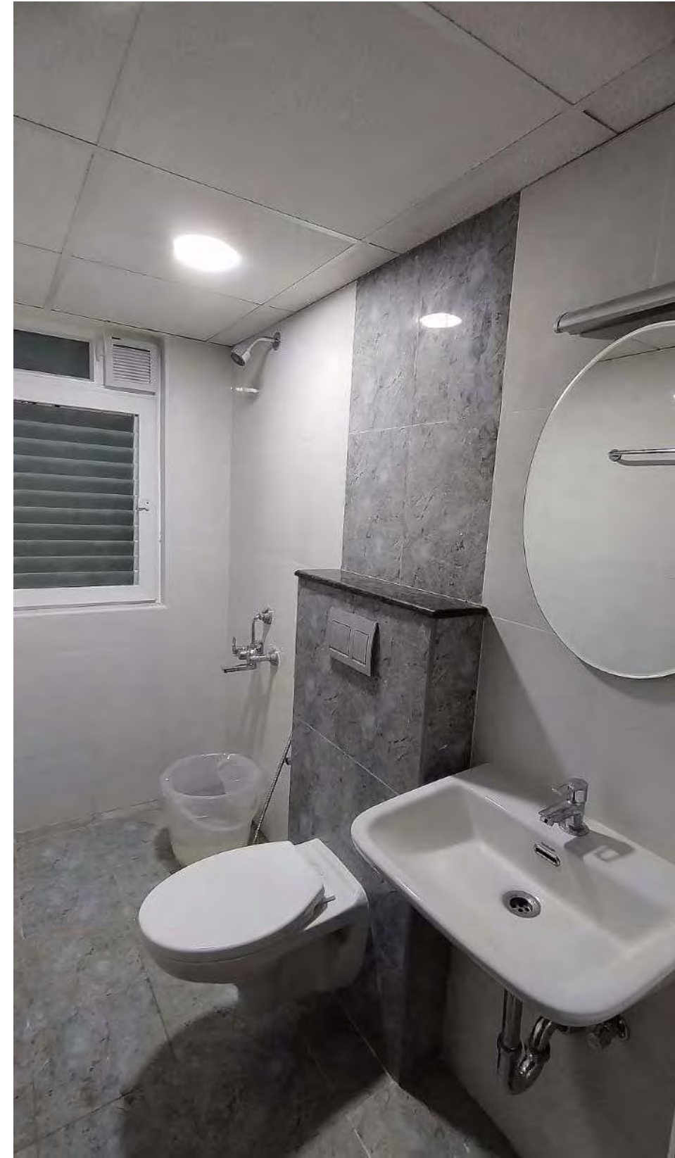
CP and Sanitary Fittings Fixing Work Completed
