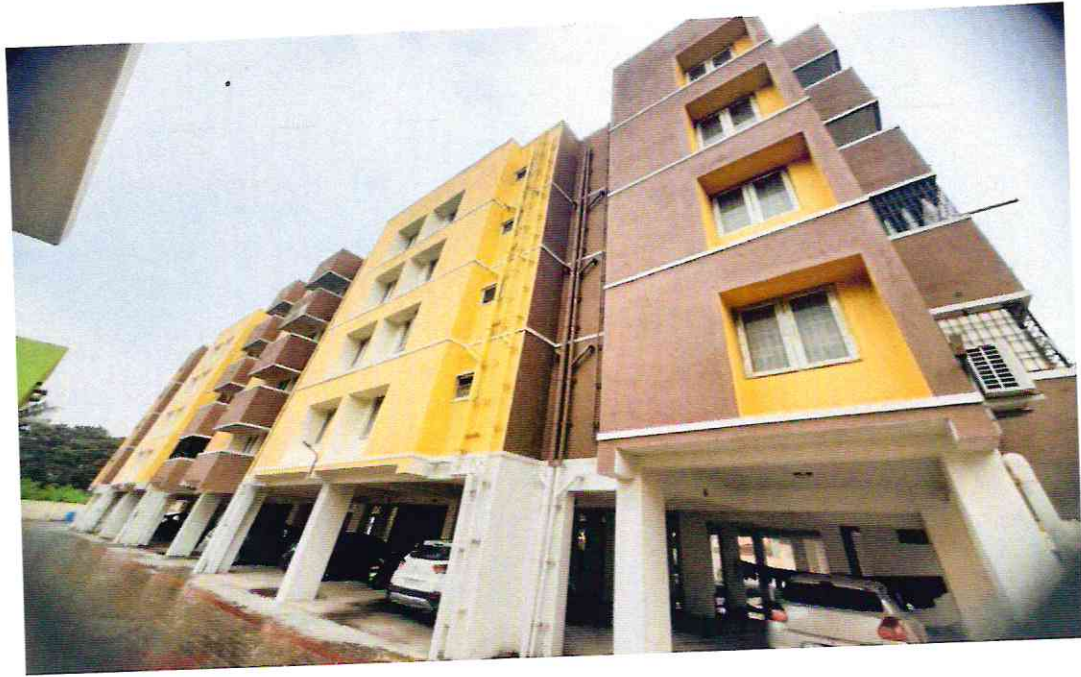
Back view - West side
