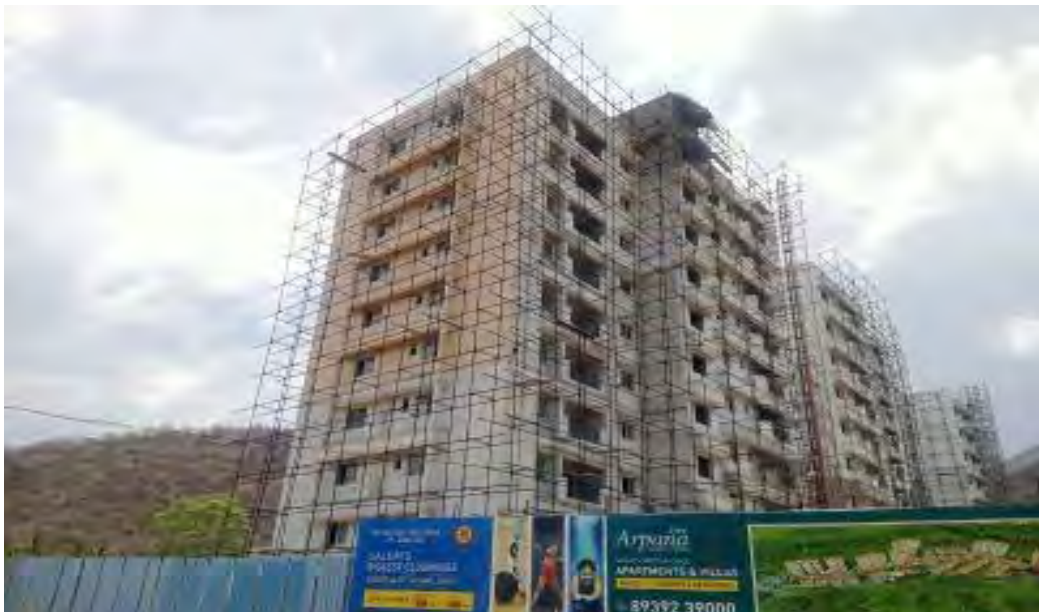
BLOCK D&E TOWER – 1 (Tower K) View -2
