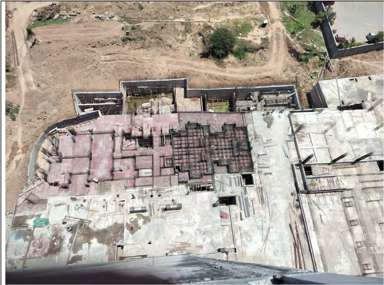
Tower 4B ground floor work in progress
