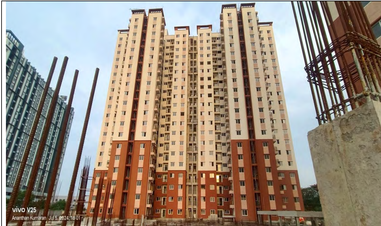
Tower 5A & 5B _ Structure completed and finishing work under progress
