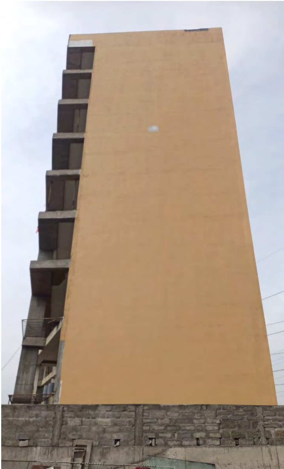
East side view as seen on 06.07.2024
