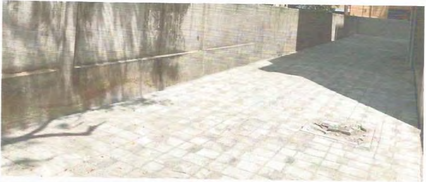
All side compound wall with gate
