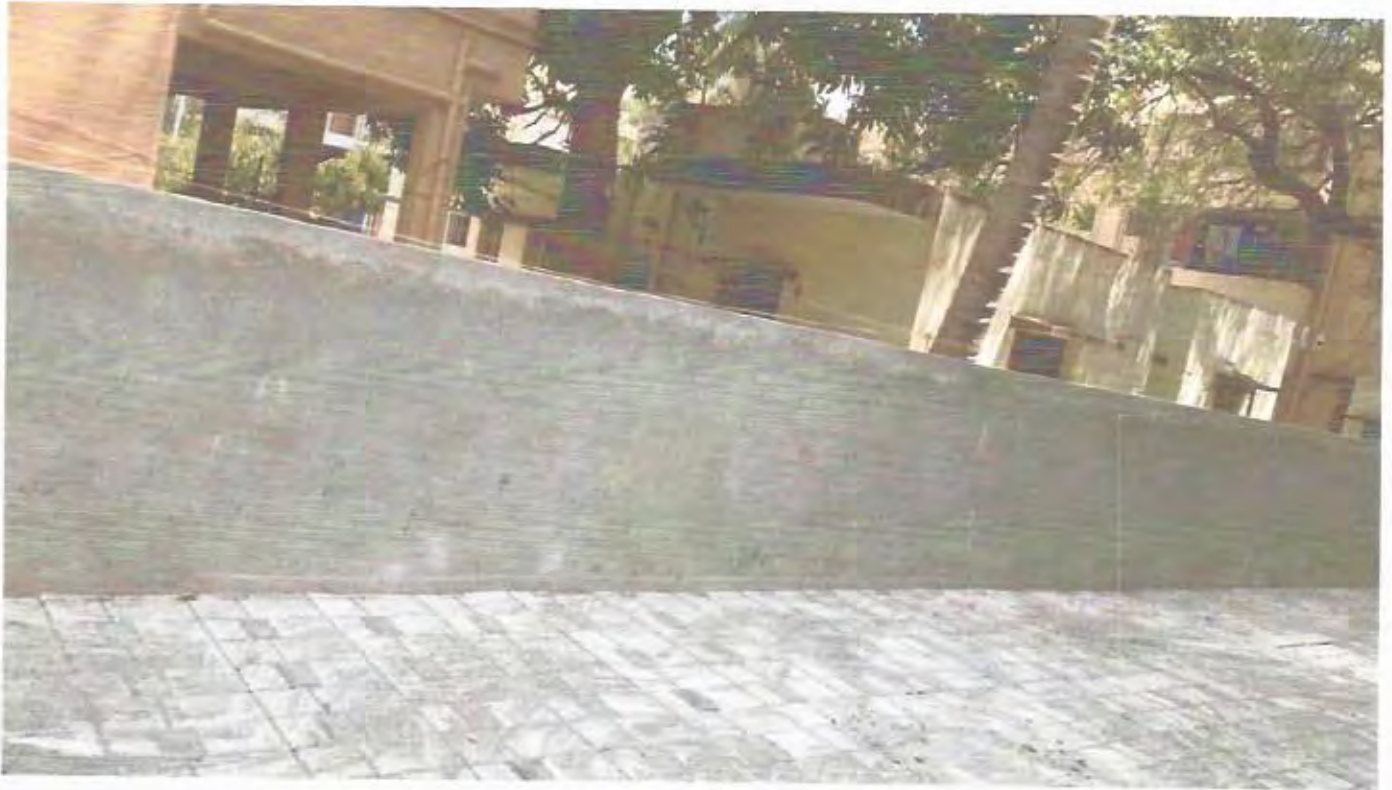
All side compound wall with gate
