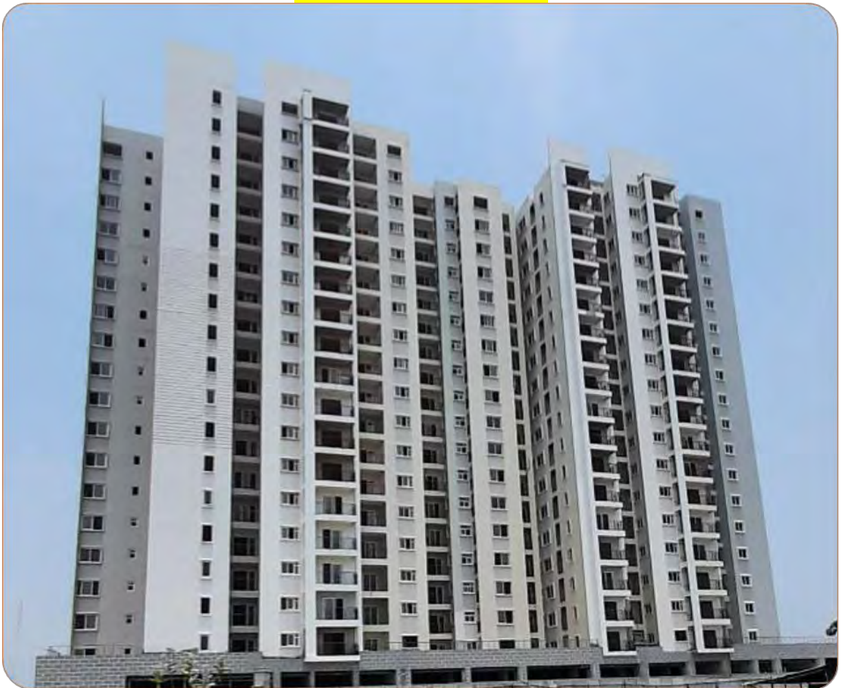
C7 Tower South Side View
