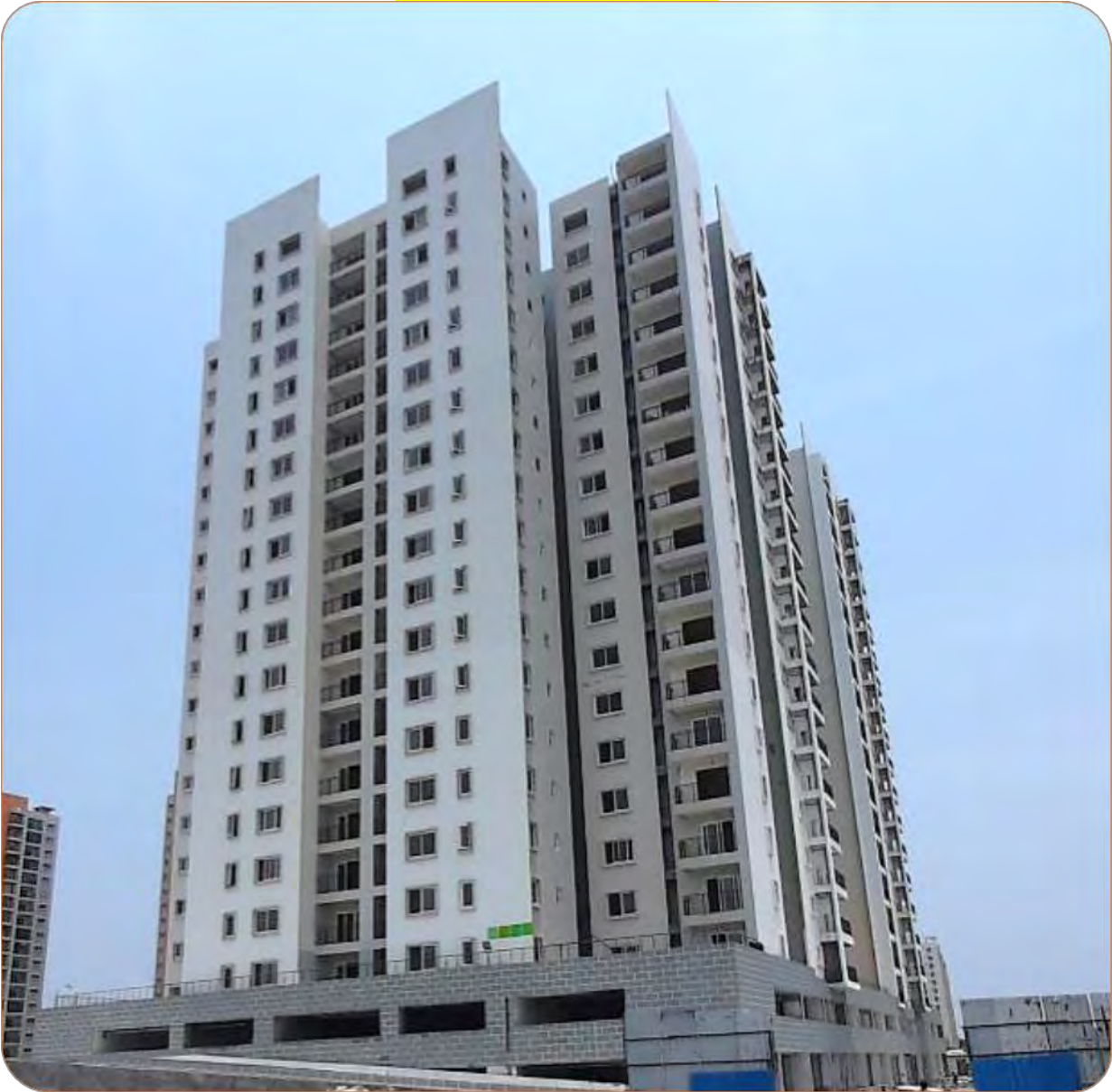
C7 Tower West Side View
